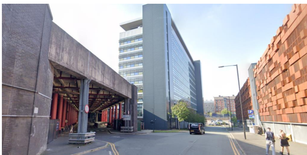
Figure 3. Parts of the listed railway station are seen amongst contemporary structures such as the above section in Sheffield Street
