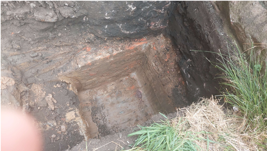
Figure 2 - Trial Pit - note foundation construction does not step out and therefore will not clash with proposed foundations
