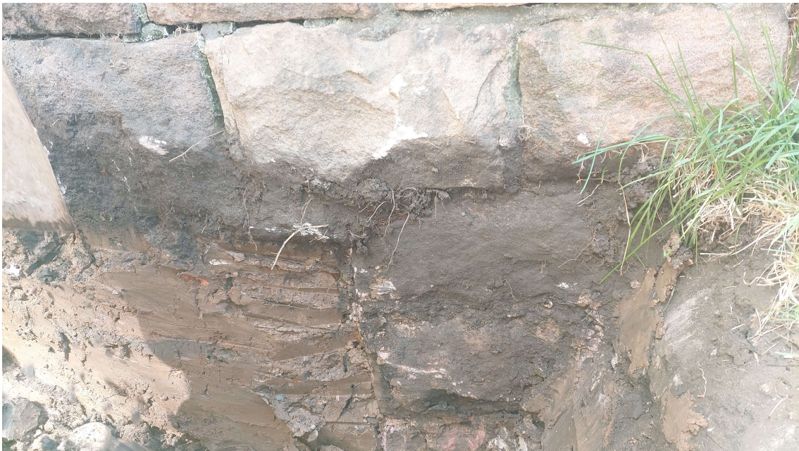
Figure 4 - Trial pit view looking at existing stairs
