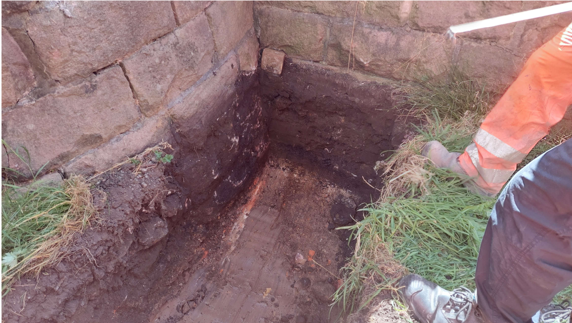
Figure 1 - Trial pit looking towards exiting stairs
