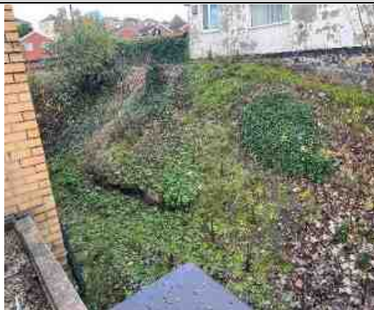
Photograph 5: Vegetated area adjacent N boundary. Steep slope down towards building's lower ground floor.
