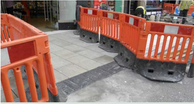
Direct access corridor from Chester Frodsham street
