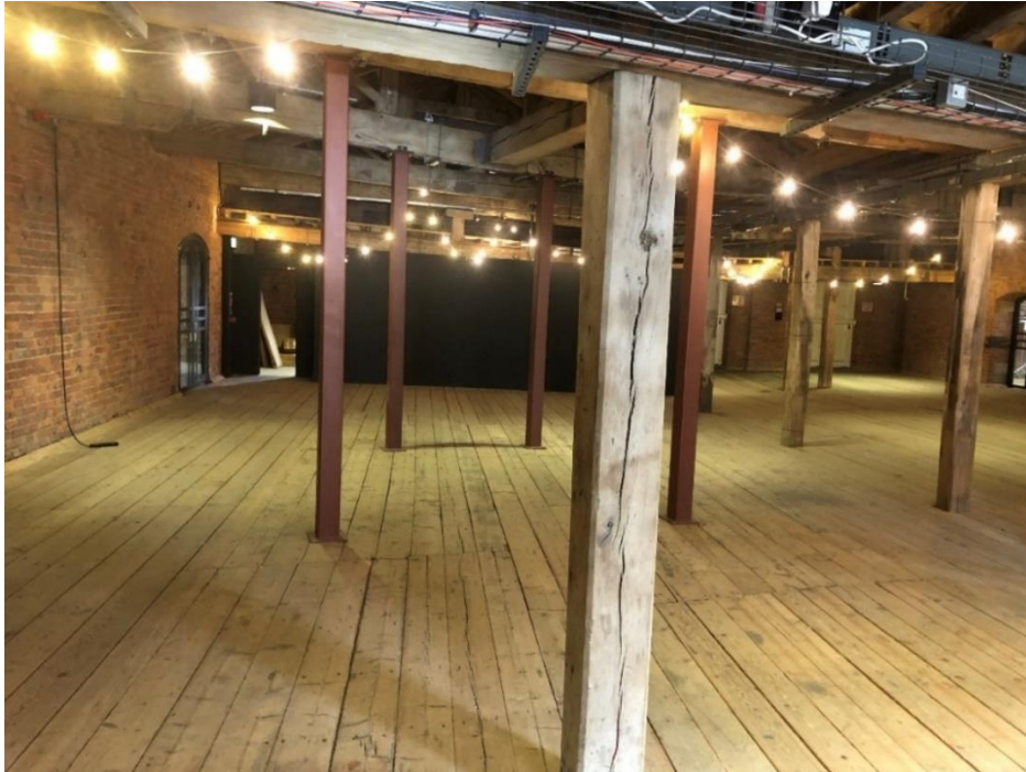
Photograph 19 – Steel props at second floor beneath roof truss ties. Note props load onto second floor beams below (i.e., they are not over columns)
