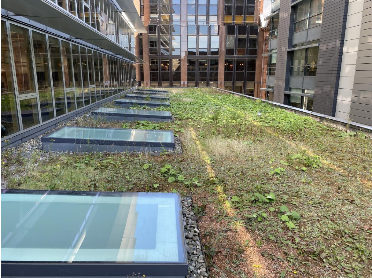
Photo 3.2 Existing second floor green roof
