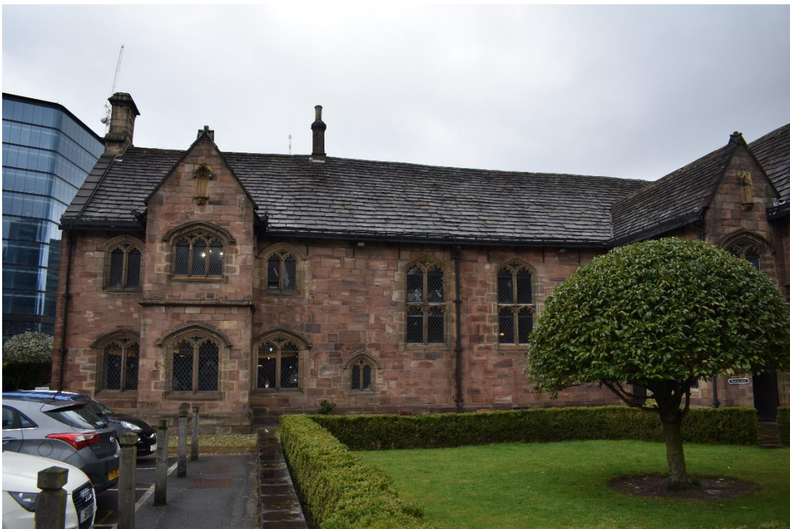
College House Baronial Hall East Elevation.
