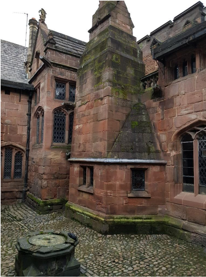
Fox's Court Well and Chimney.
