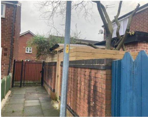
Canopy at the rear of the dwelling
