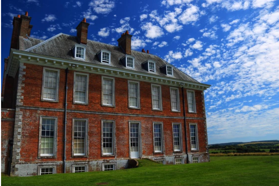
Figure 2 – Uppark, Suffolk, showing the use of a sash window-door to the centre of the rear elevation, allowing for the fenestration pattern to remain unaltered.
