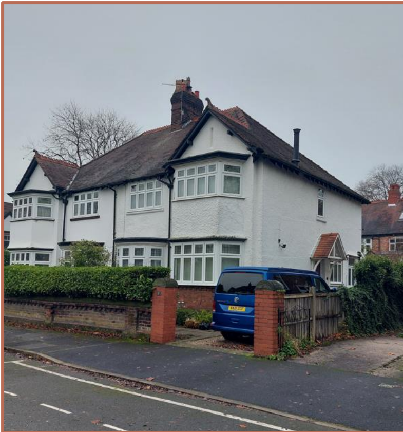
Figure 2: Photograph showing 3 St Aldwyns Rd: December 2022
