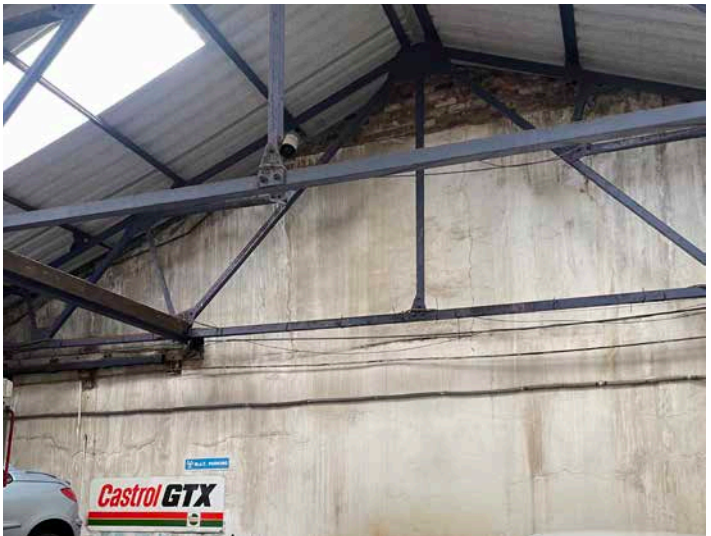
North West elevation seen from garage internally. Rendered.
