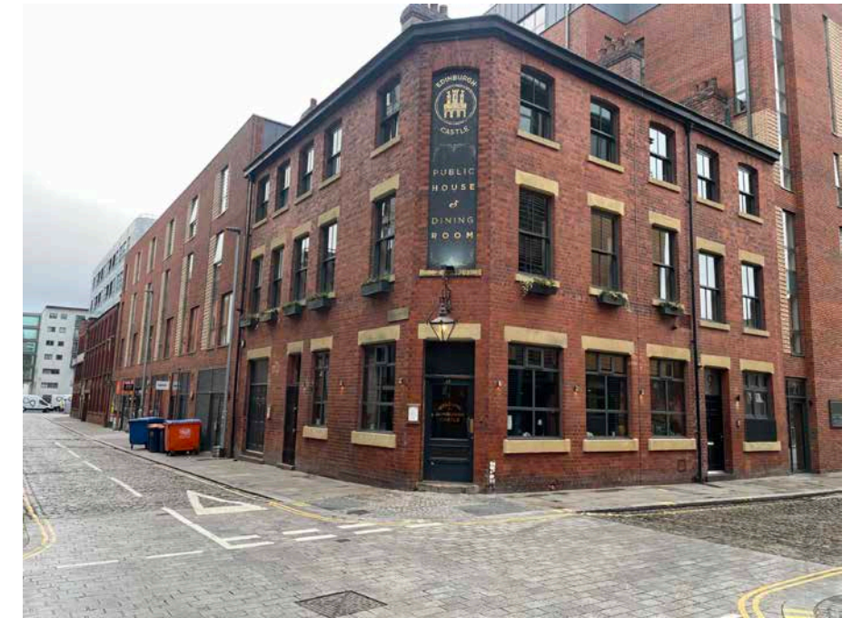
Historic Edinburgh Pub, residential use to upper floors.
