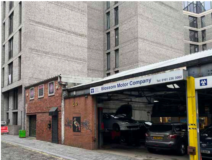
Henry Street frontage, slight views of side elevation.
