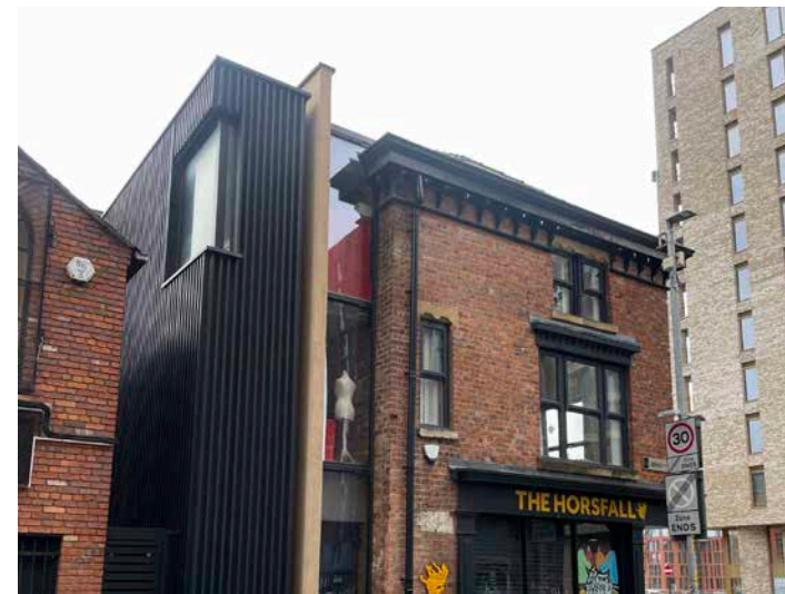
Contemporary extension to the former Coates School
