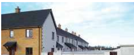
Social Housing Installation Co. Louth, Ireland
