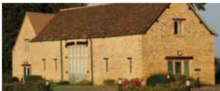
Barn Conversion Wing, England
