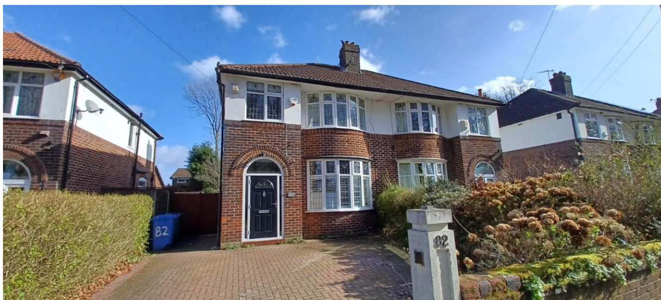
Figure 1. Principal elevation of No.82 Parkville Road.
