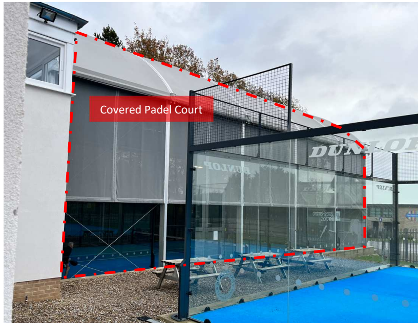
Figure 3.1: Covered Padel Court assessed in measurements
