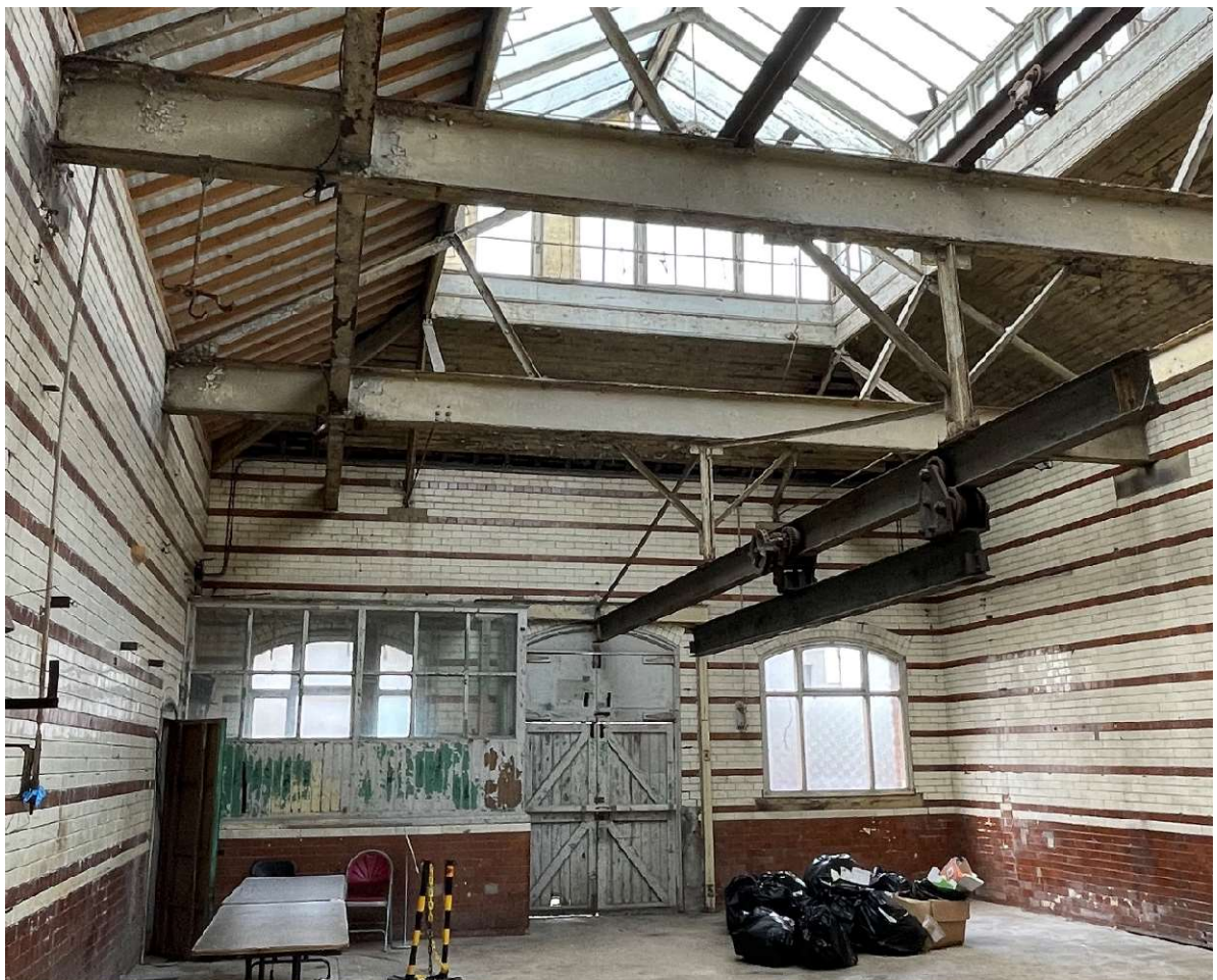
Interior of the Laundry Looking west
