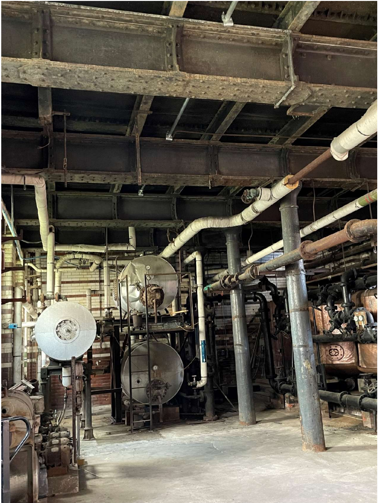
Plant rooms to the north of the Females Pool
