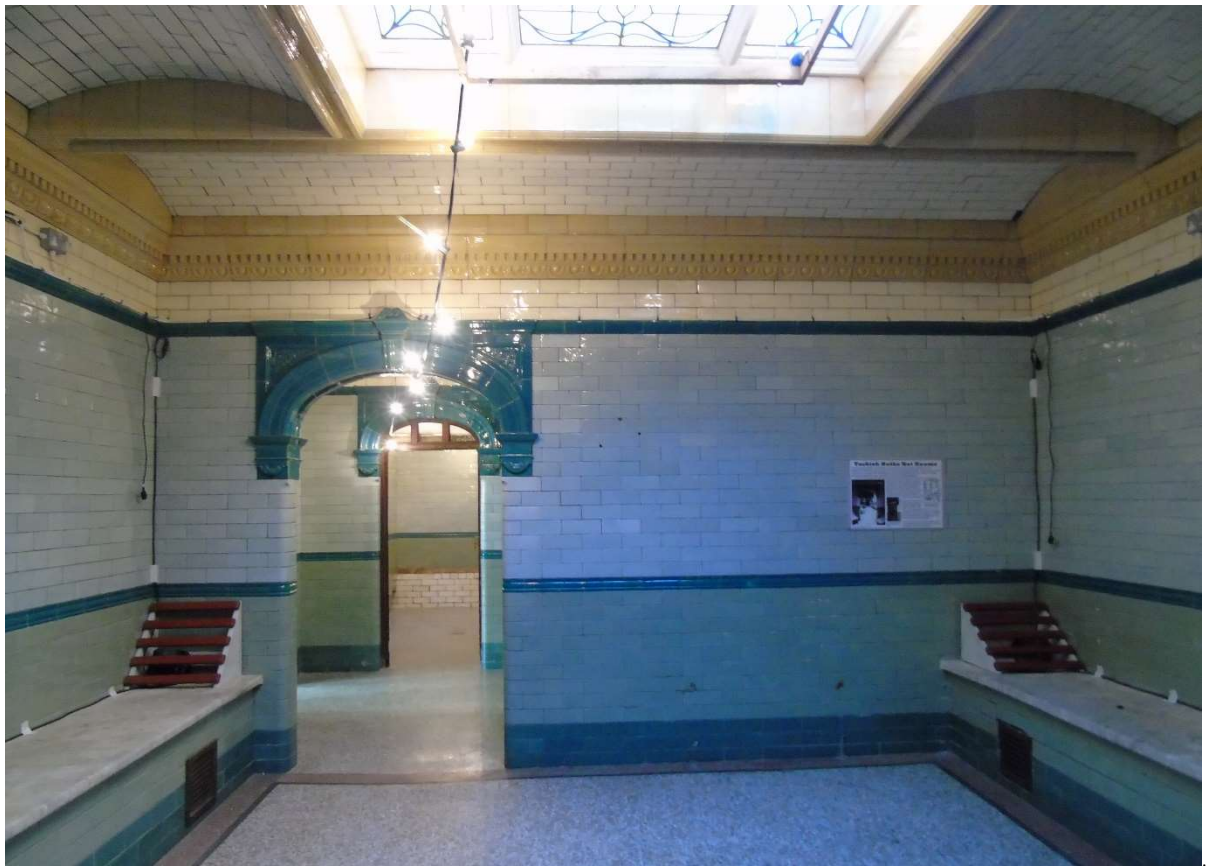
Fully tiled rooms including ceilings with laylights
