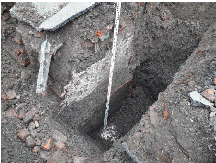
Brick wall visible in north western wall of pit and concrete floor visible.
