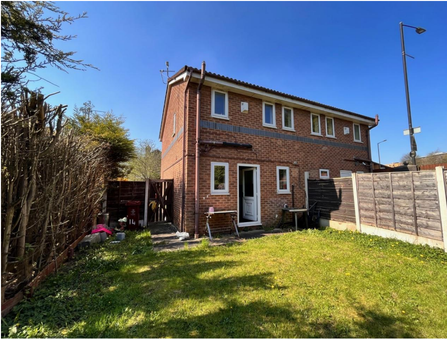
View of property as existing from the rear
