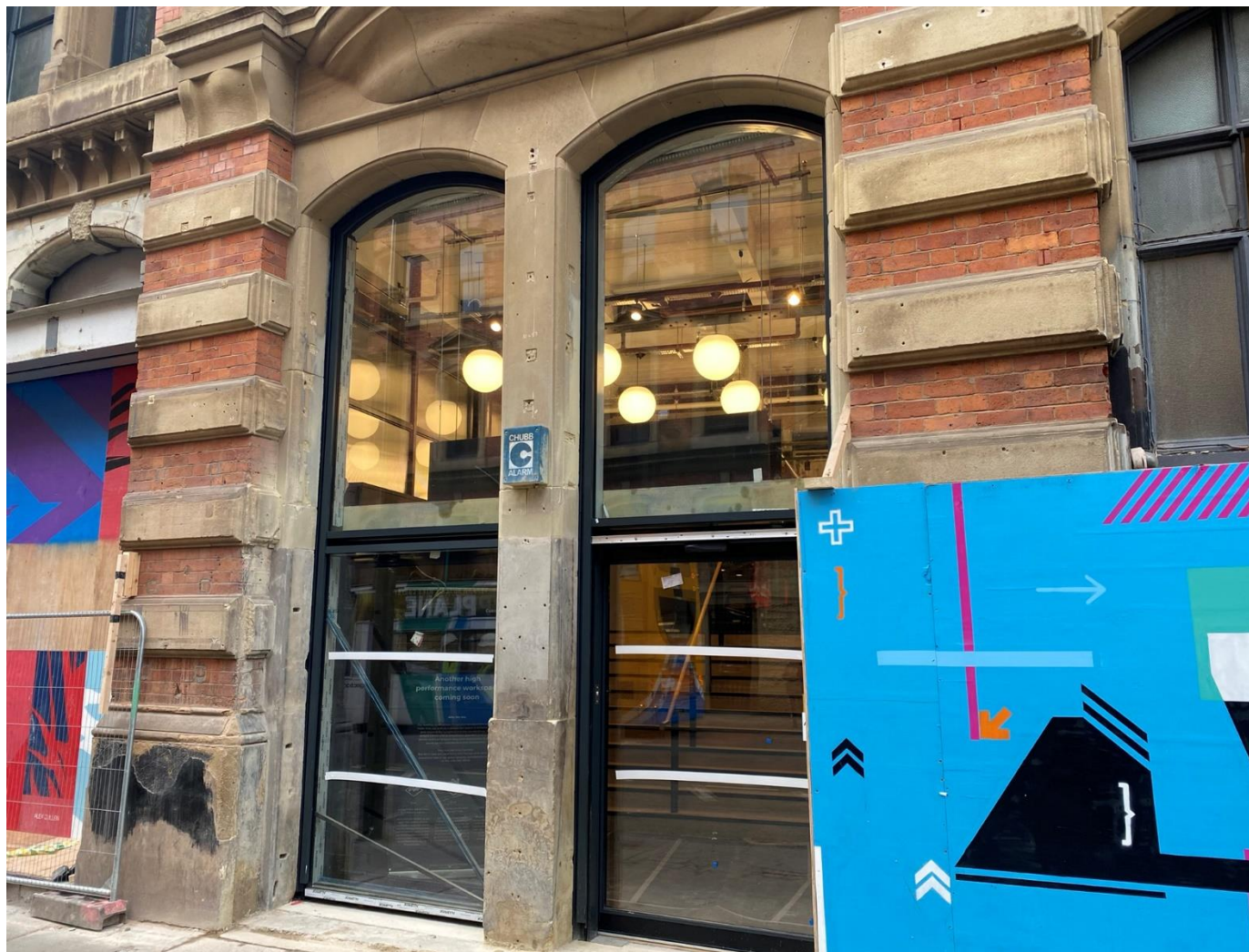
Current photograph taken during construction phase showing redundant alarm box and ongoing stone repairs to central stone column
