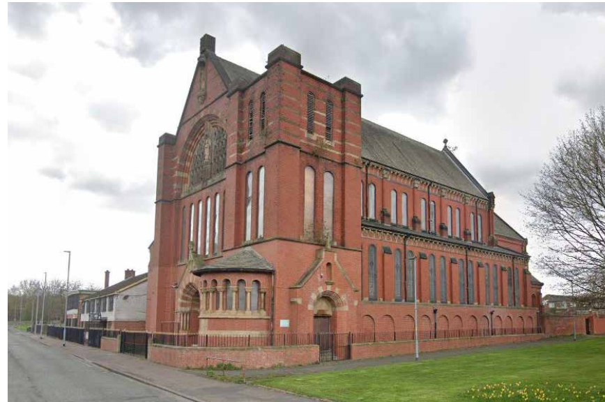
Usmania Banqueting Hall
