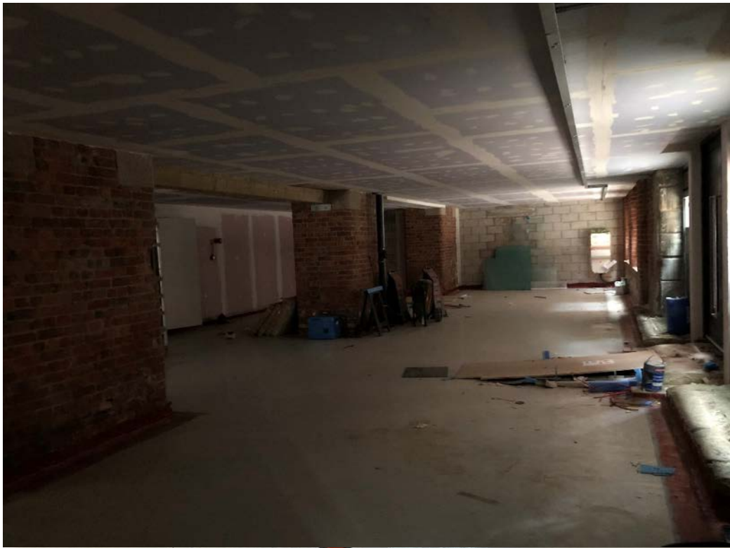
03 view of unit existing interior
