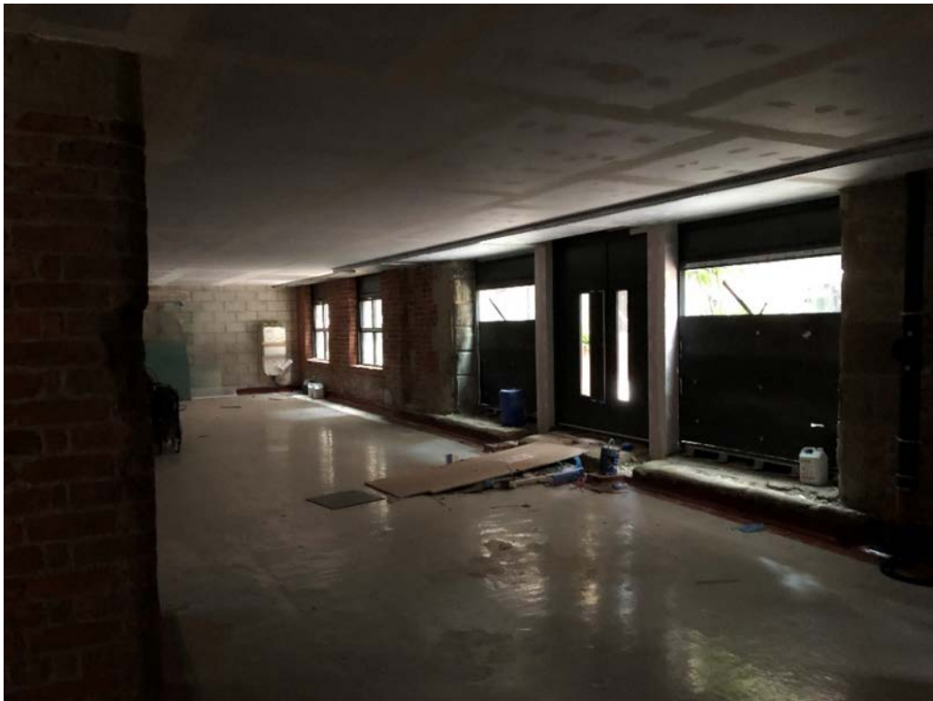
04 view of unit existing interior
