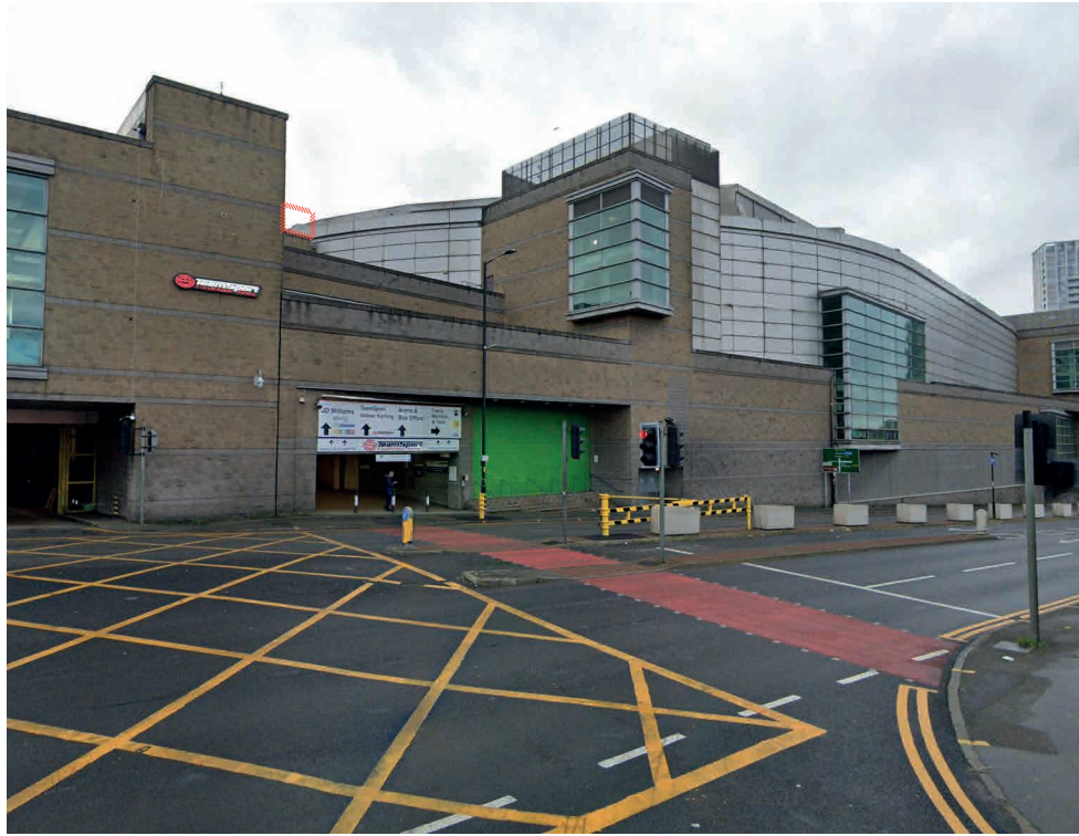
Existing view from Trinity Way looking towards the Trinity Tunnel
