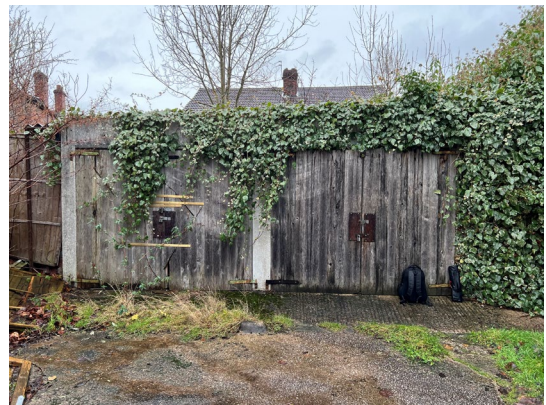
Existing dilapidated garage block
