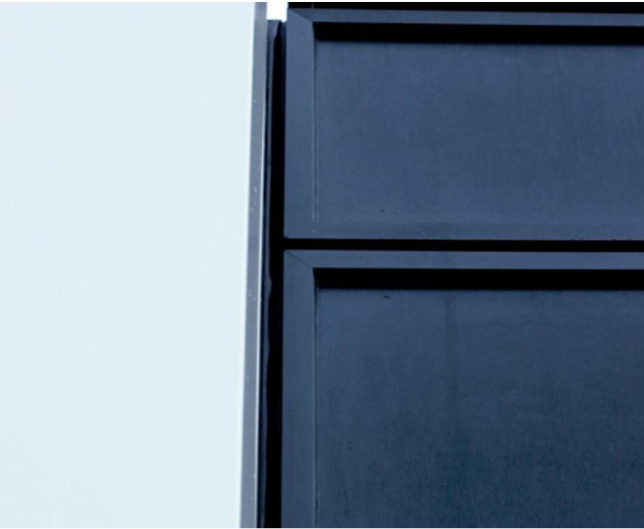
Figure 3: Unitised panel interface for Vita T1
