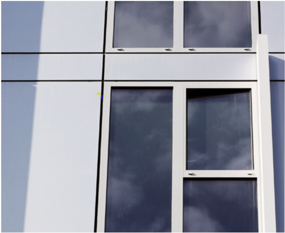
Figure 4: Unitised panel interface for Trinity Riverview
