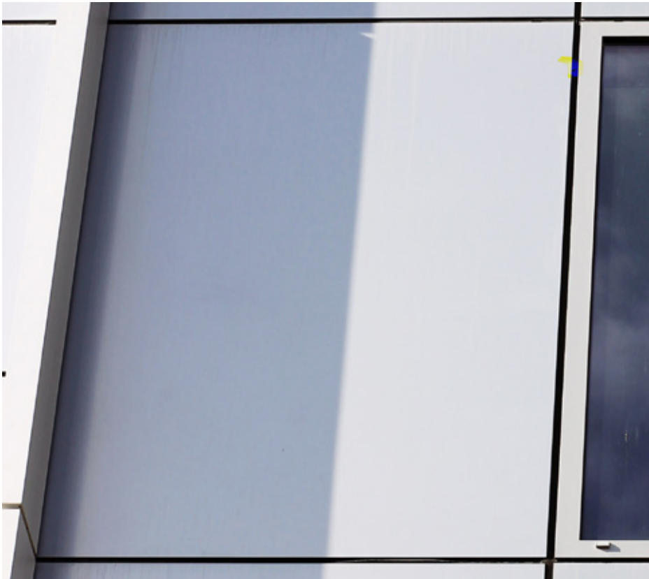
Figure 6: Standard black gaskets between facade panels
