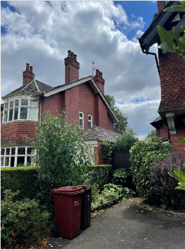
Front / western side elevation of 322 Lapwing Lane towards no. 320 Lapwing Lane
