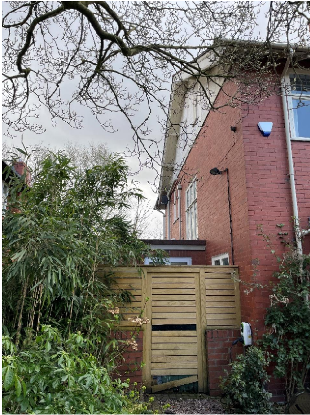
Eastern side / front elevation with existing flat roofed side extension behind gated screen fencing.
