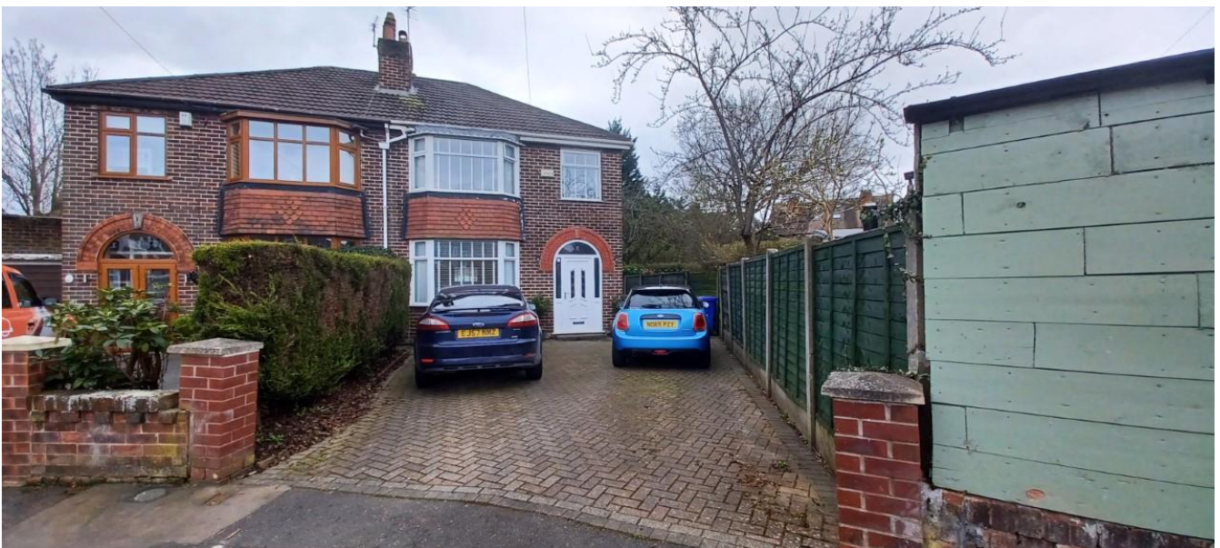
Figure 1. Principal elevation of No.2 Rangemore Avenue.
