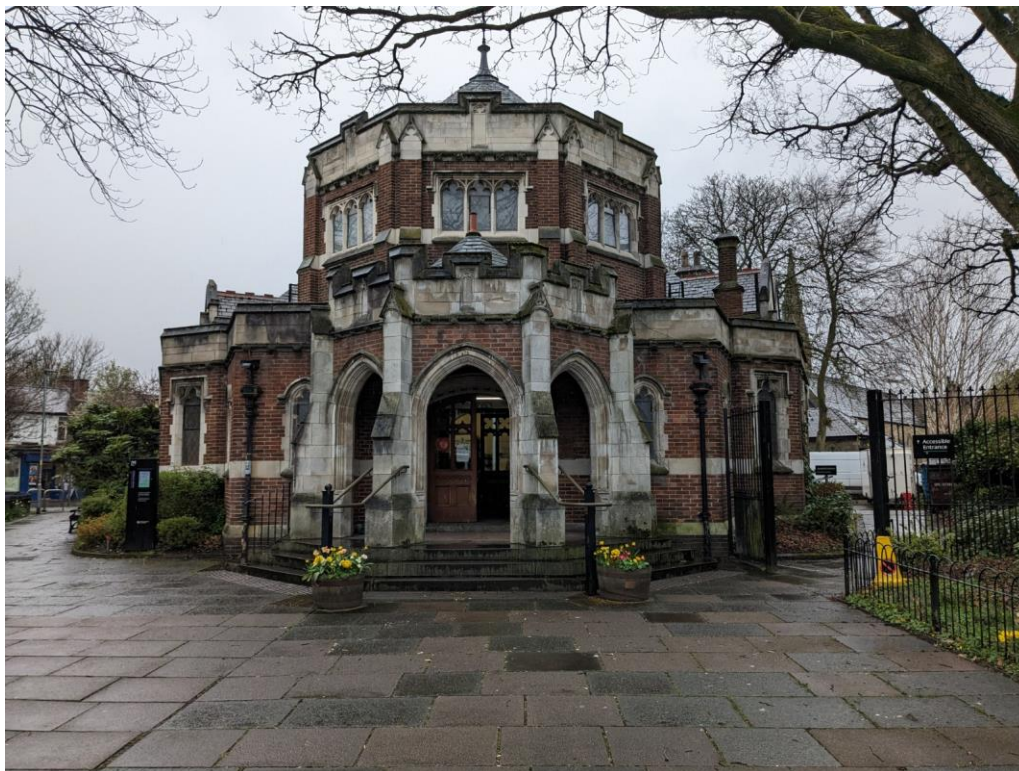
Didsbury Library – Wilmslow Road Frontage
