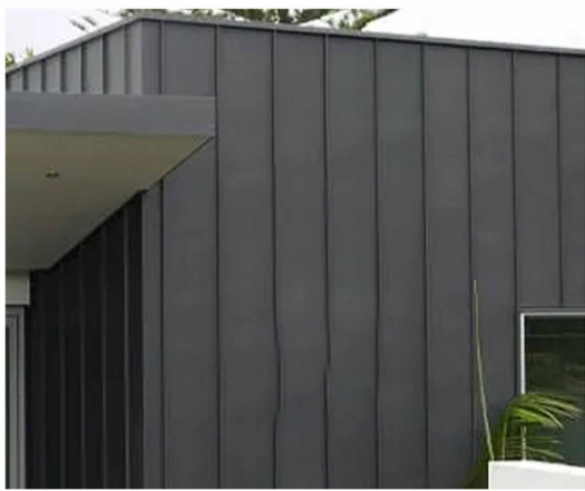
2 Viero Vertically Laid Standing Seam Built-up Cladding System
