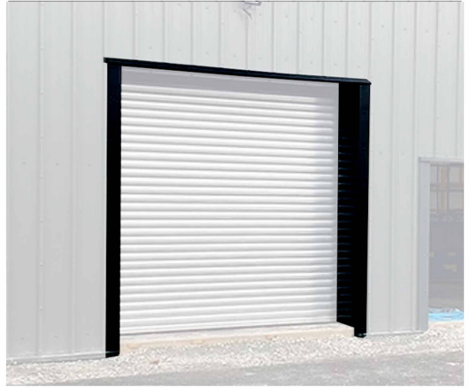
10 Feature Projecting Portico Over Loading Doors Material - Pressed Metal Finish
