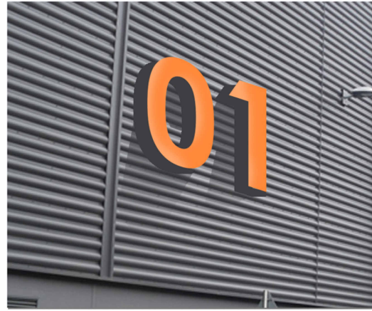
12 PPC Aluminium Unit Identification Numbering To Specialist Sub-Contractor Design Size - Height 1350mm | Depth 150mm
