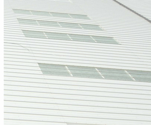
8 Rooflight System integrated compatible with roof cladding system
