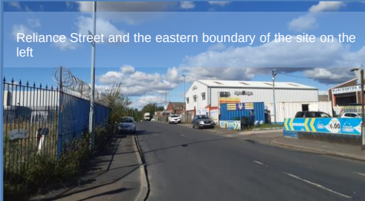
A view across the site from Reliance Street towards the apartment building 53 Ivy Green Close
