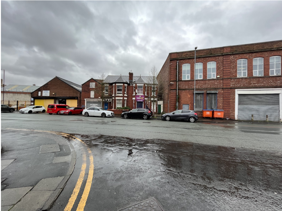
Image 2: West elevation of buildings 1, 2 & 3.
