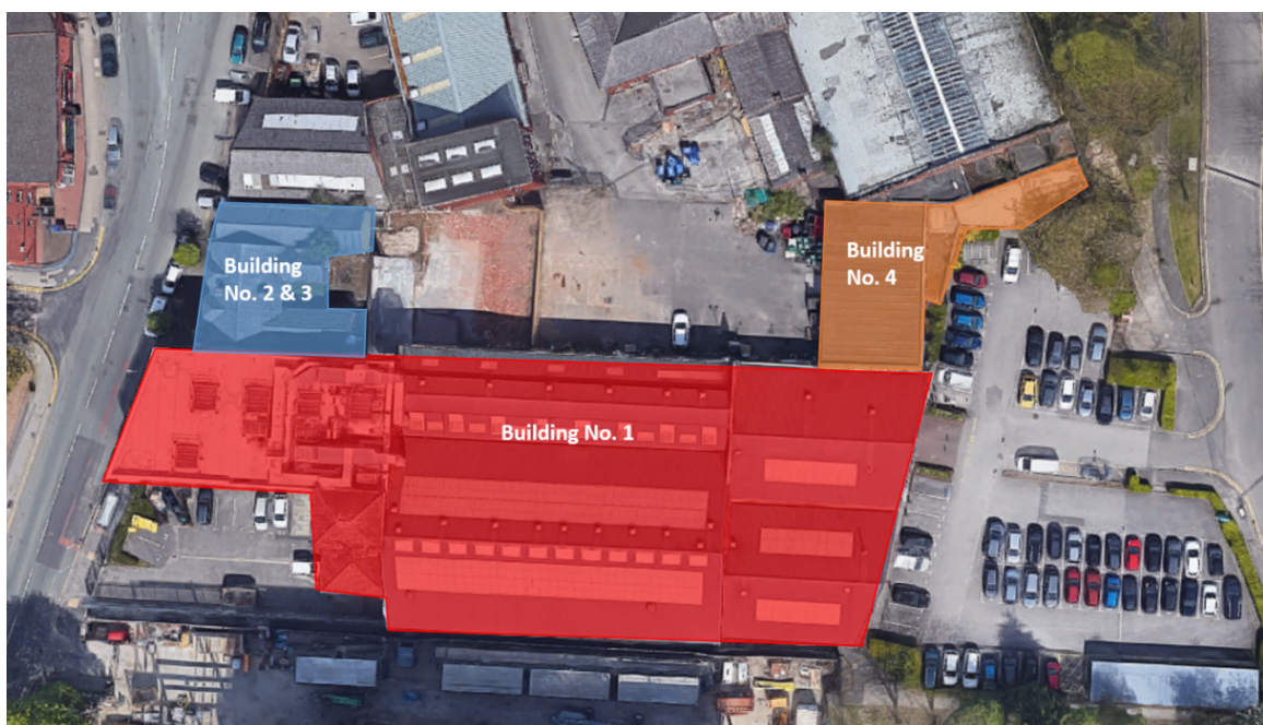
Fig5: Overview of buildings scheduled for demolition.
