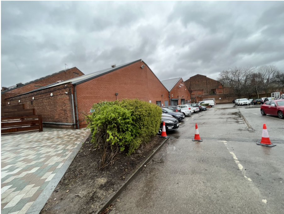
Image 4: South-east section of building 1 and adjacent car park (within demolition site).
