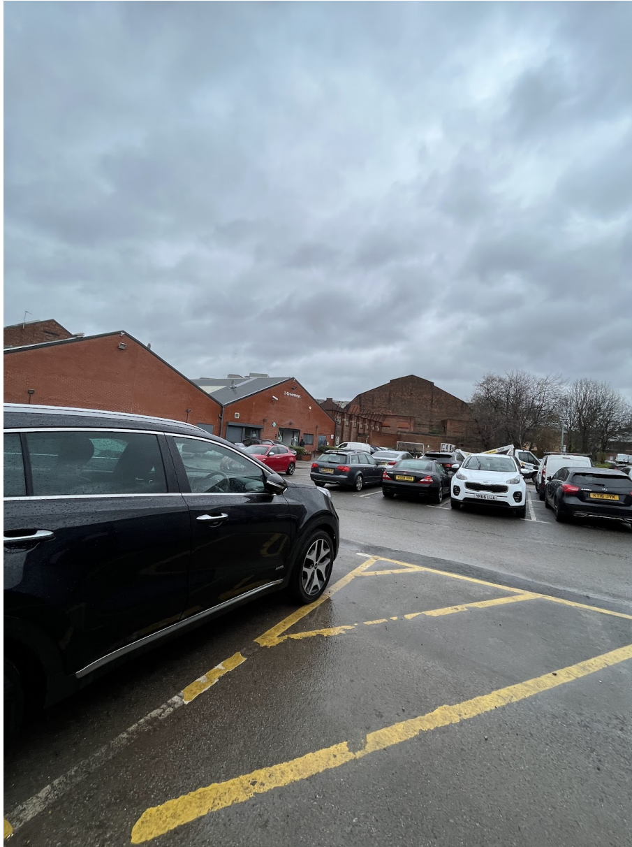
Image 5: East elevation of building 1. East elevation of building 4 visible in back ground.
