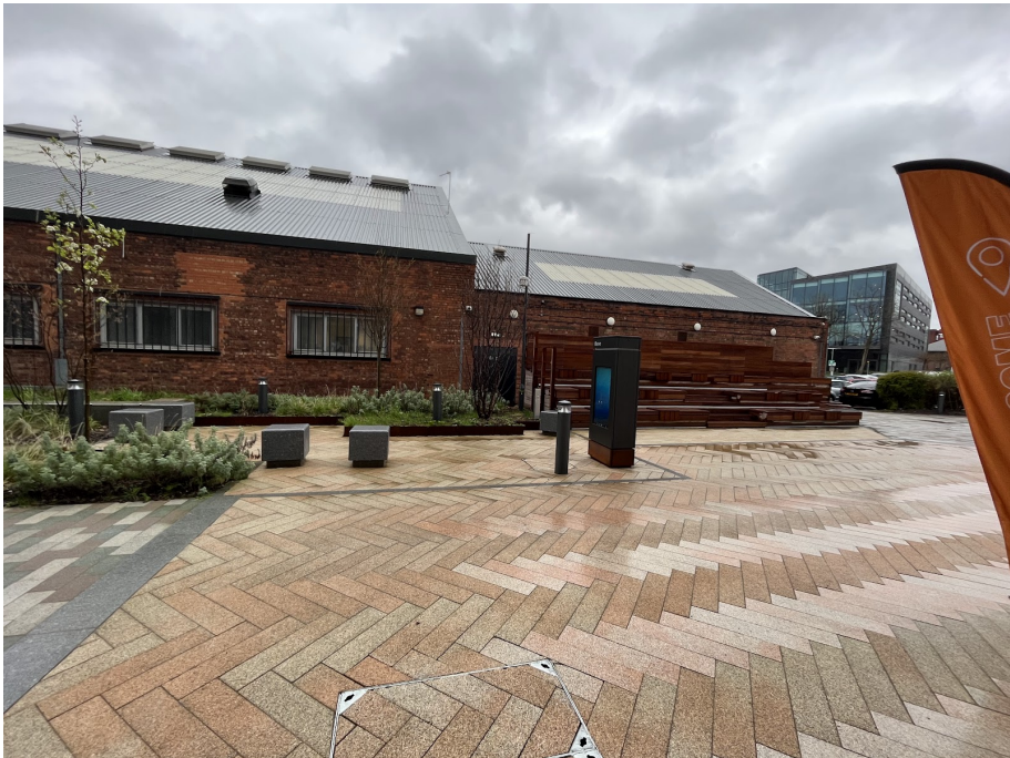
Image 8: South elevation (eastern portion) of building 1.
