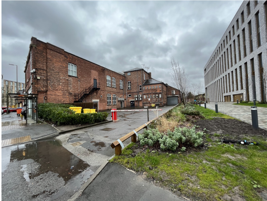
Image 6: Service yard in west section of building 1.
