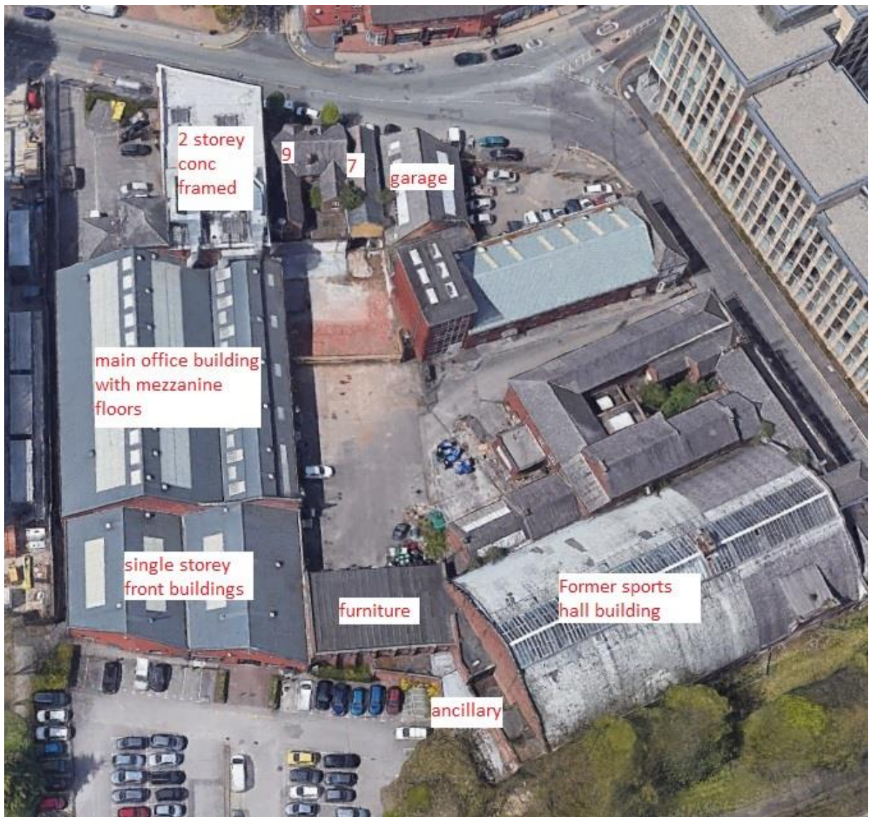
Aerial view from East indicating structures to be demolished and the Garage and Sports Hall buildings that are to remain occupied during the works
