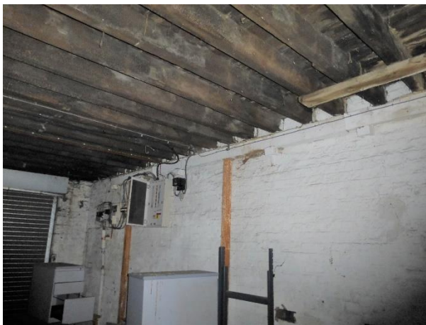
Underside of first floor joists
