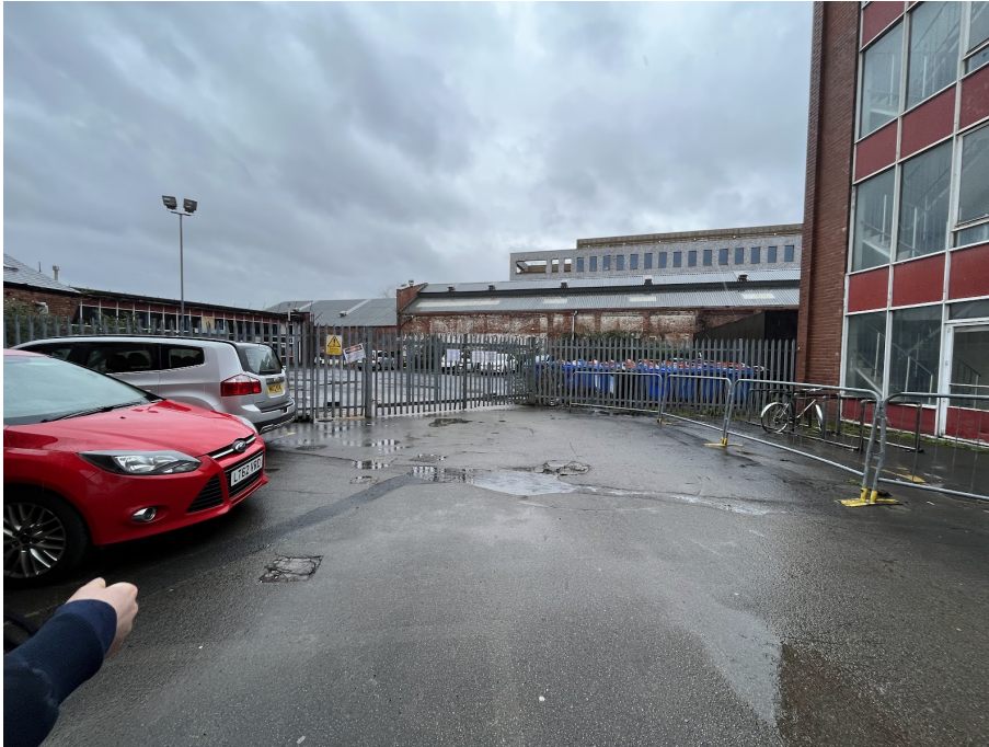
Image 3: North elevation of building 1 and west elevation of building 4 visible behind fencing.
