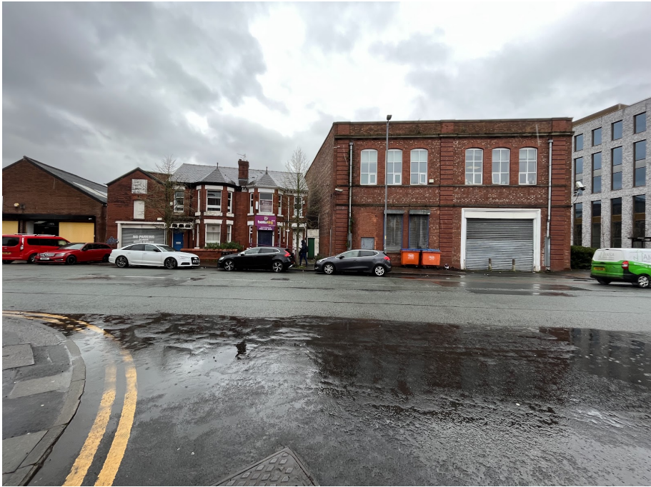
Image 1: West elevation of buildings 1, 2 & 3.
