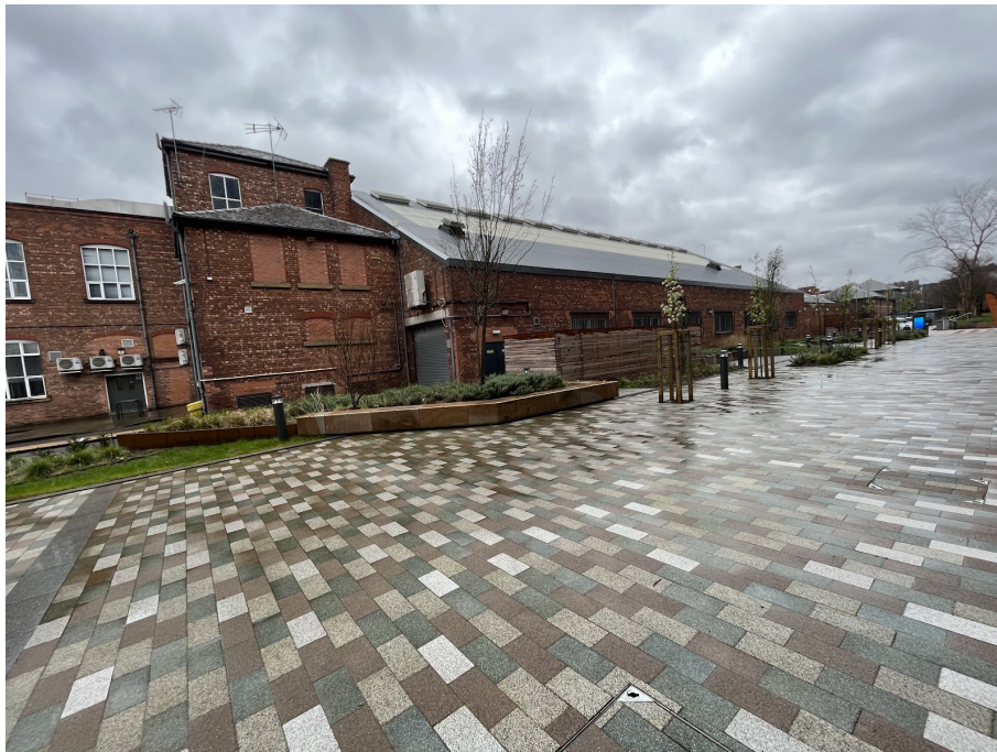
Image 7: South elevation of building 1.
