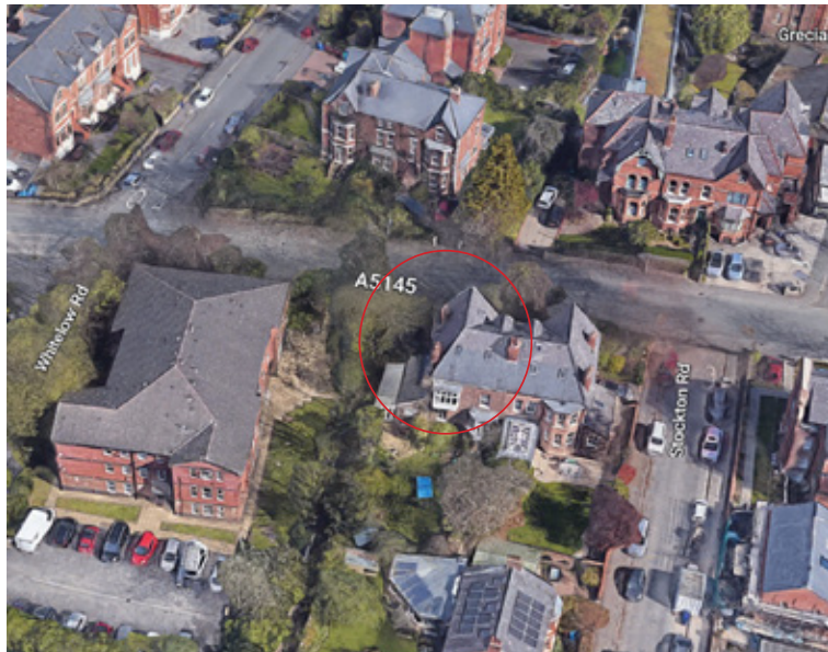
63 High Lane from the south
