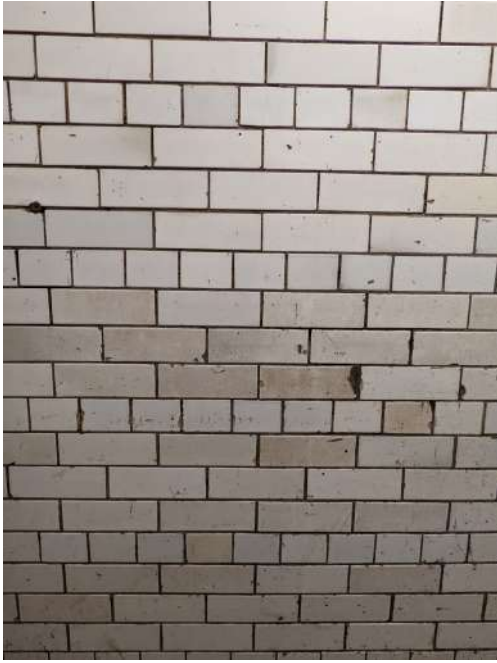
Glazed brick wall retained
