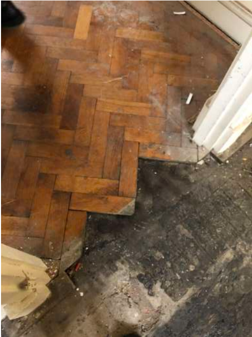
Parquet relocated within building
