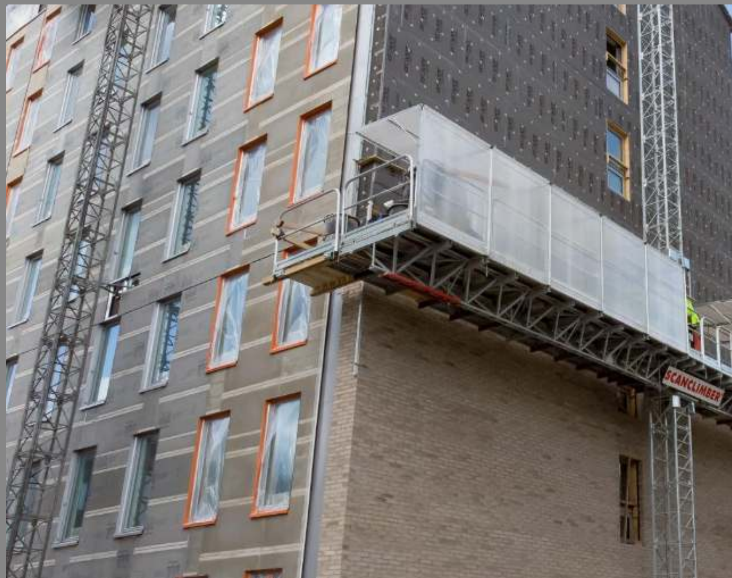
Typical mast climber protection netting to protect against material falling onto waterway
