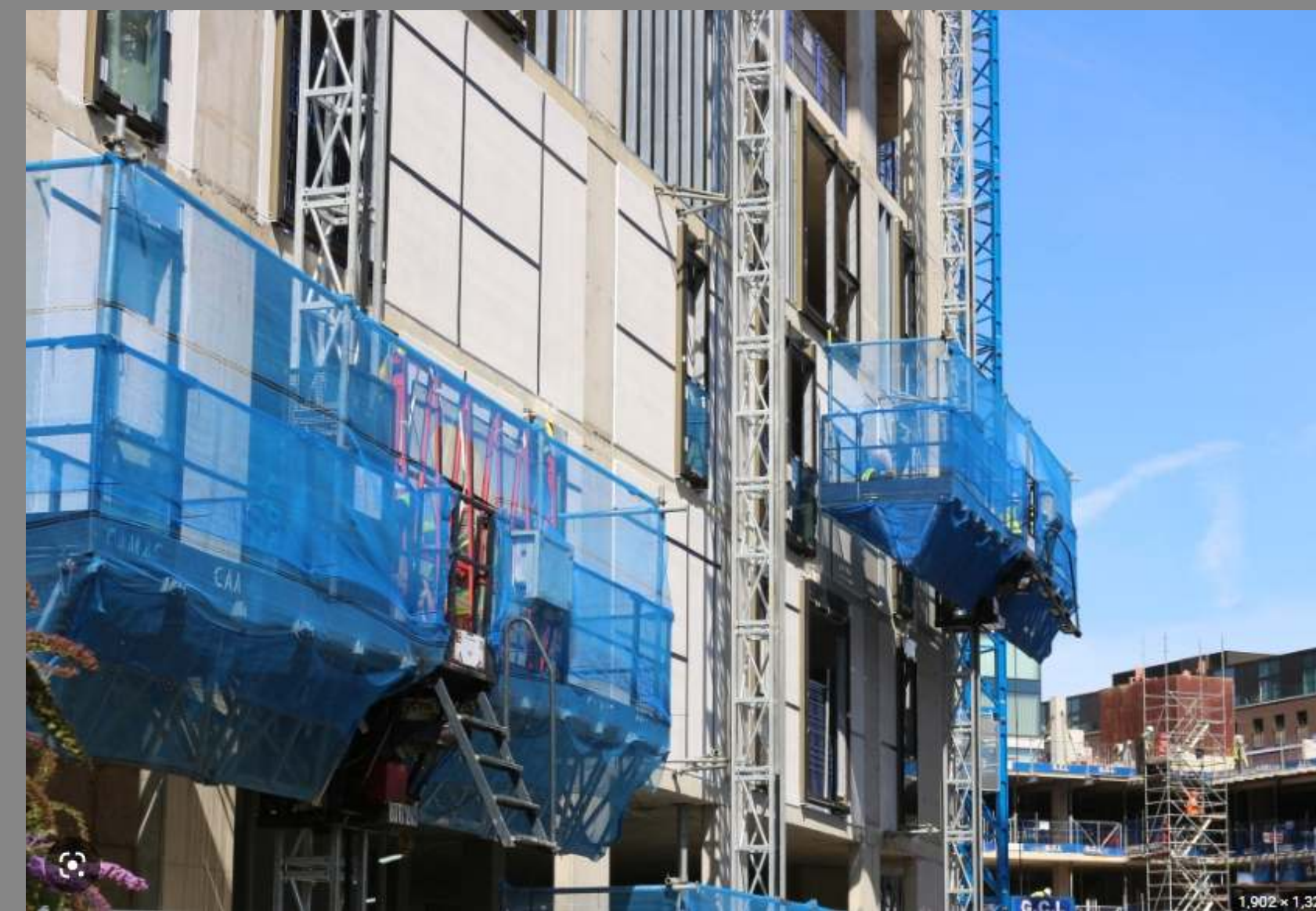
Typical mast climber protection netting to protect against material falling onto waterway
