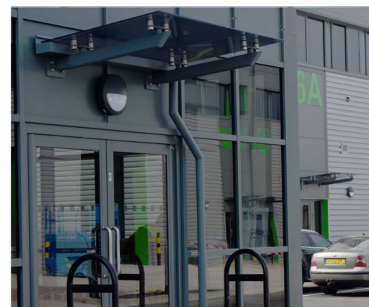
11 Glazed Canopy Over Main Entrance Frame
