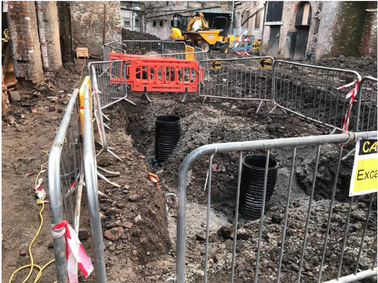
Courtyard: Manhole construction
