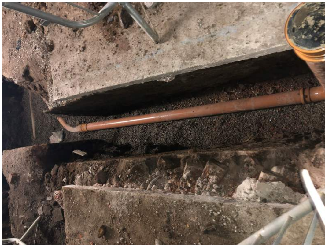
Building 2: internal drainage
