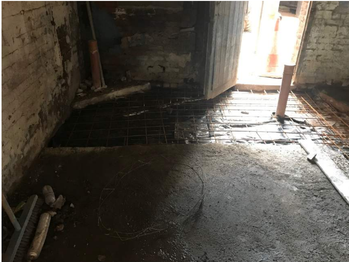
Floor reinstatement, after drainage
