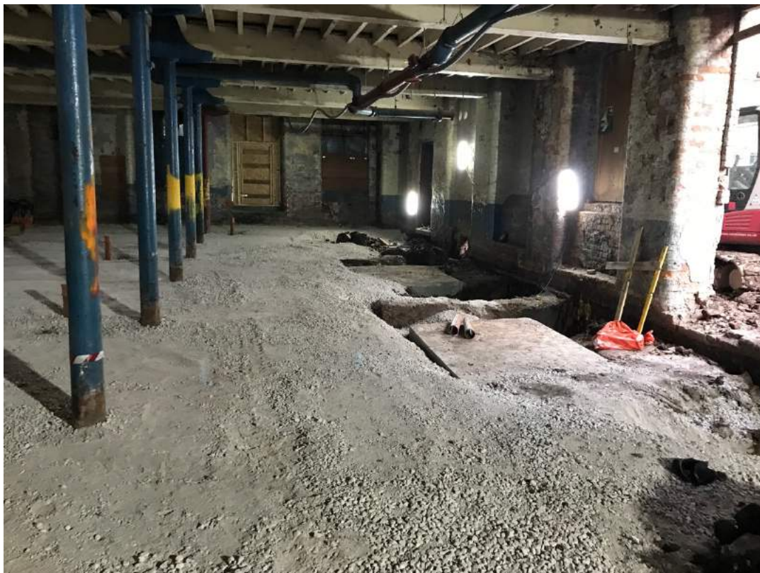
Building 2: formation after drainage
