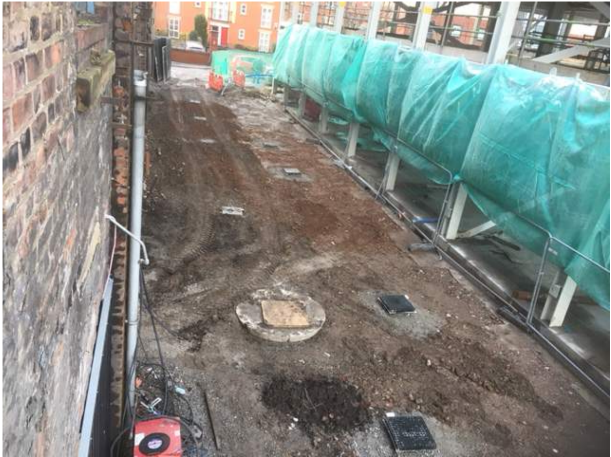
Completed drainage to East elevation of the building
