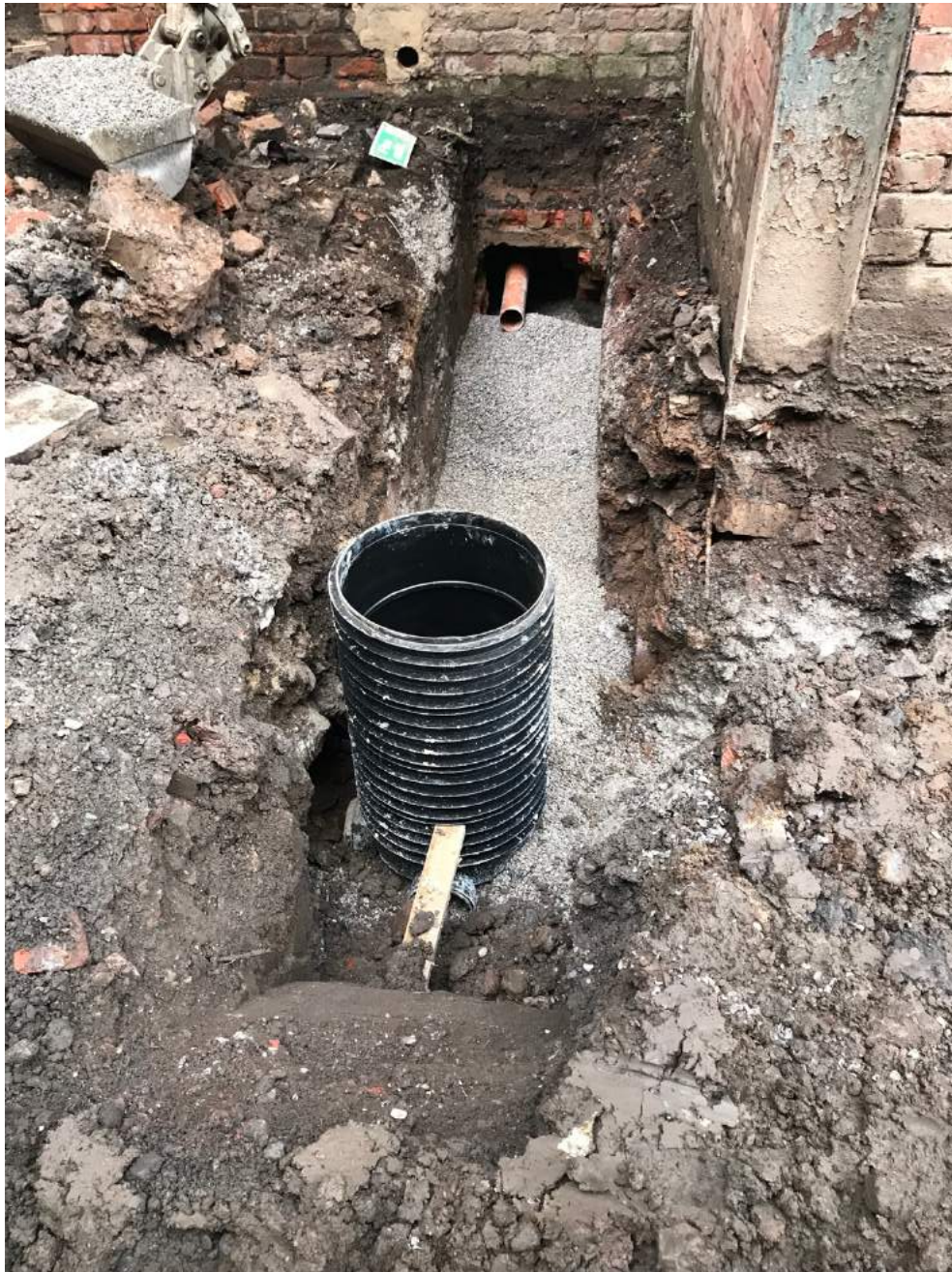
Building 2: drainage connection to manhole
