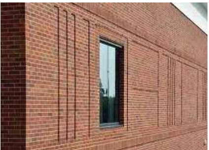
RECESSED BRICKWORK PANEL
