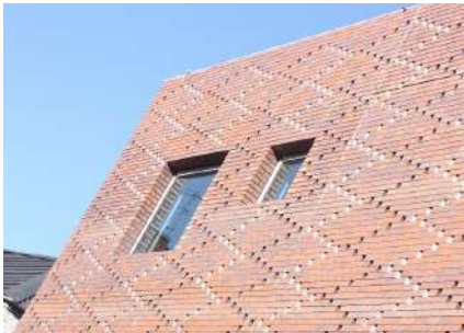
CROSSHATCH RECESSED BRICKWORK DETAIL
