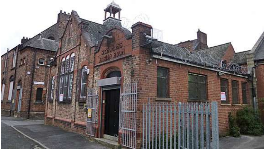
3. Parish Rooms to the North
