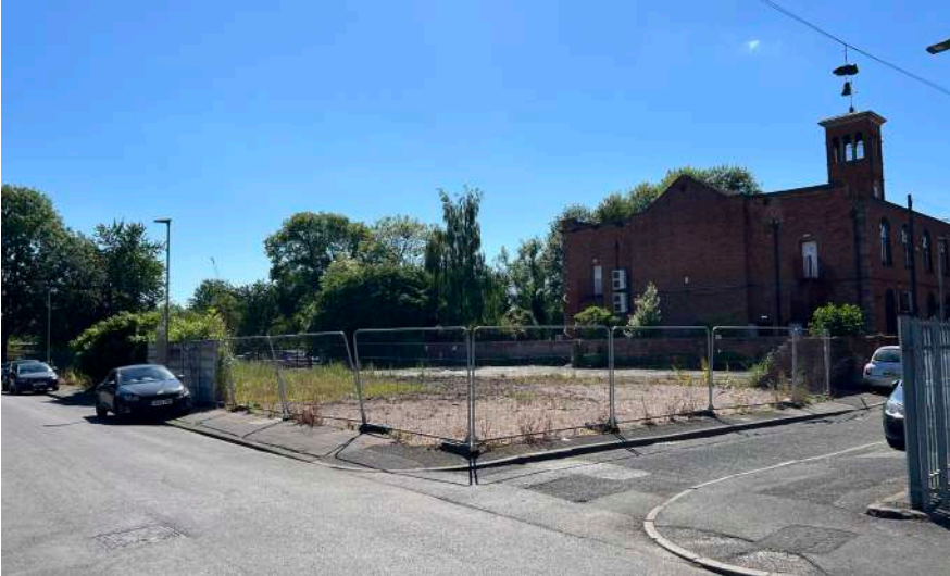
2. View of the North West corner of the site
