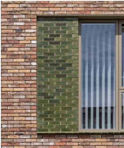
CROSSHATCH RECESSED BRICKWORK DETAIL
