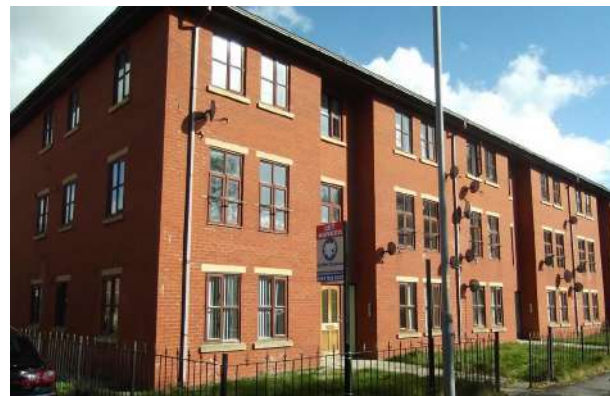
Apartments along Ardwick Road North
