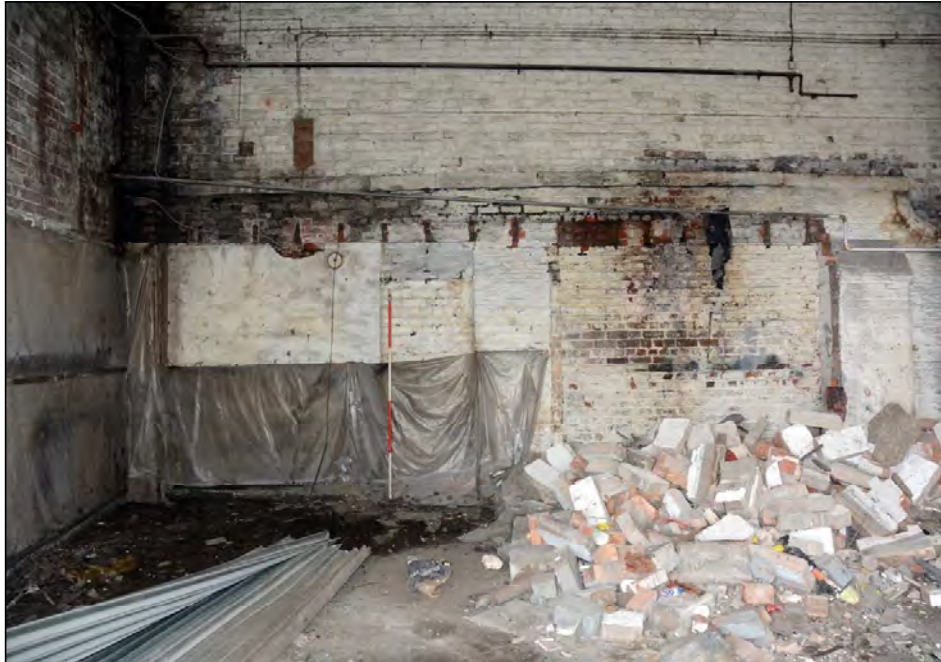
Plate 7. Wall scars of inserted floor or loft in The Warehouse, looking south
