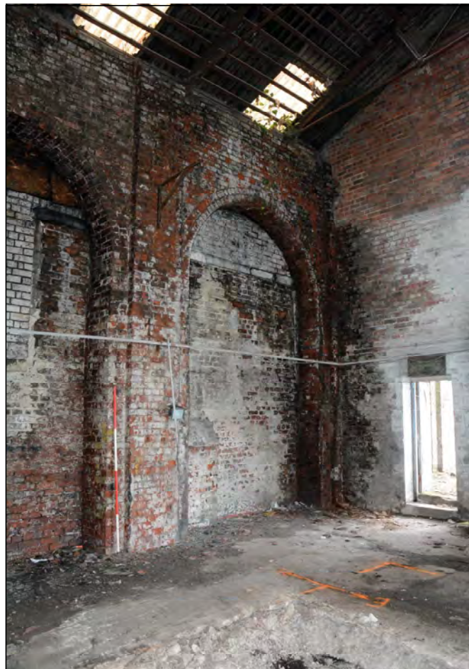
Plate 12. Detailed view of an arch of The Warehouse with other phases of walling, looking north-west
