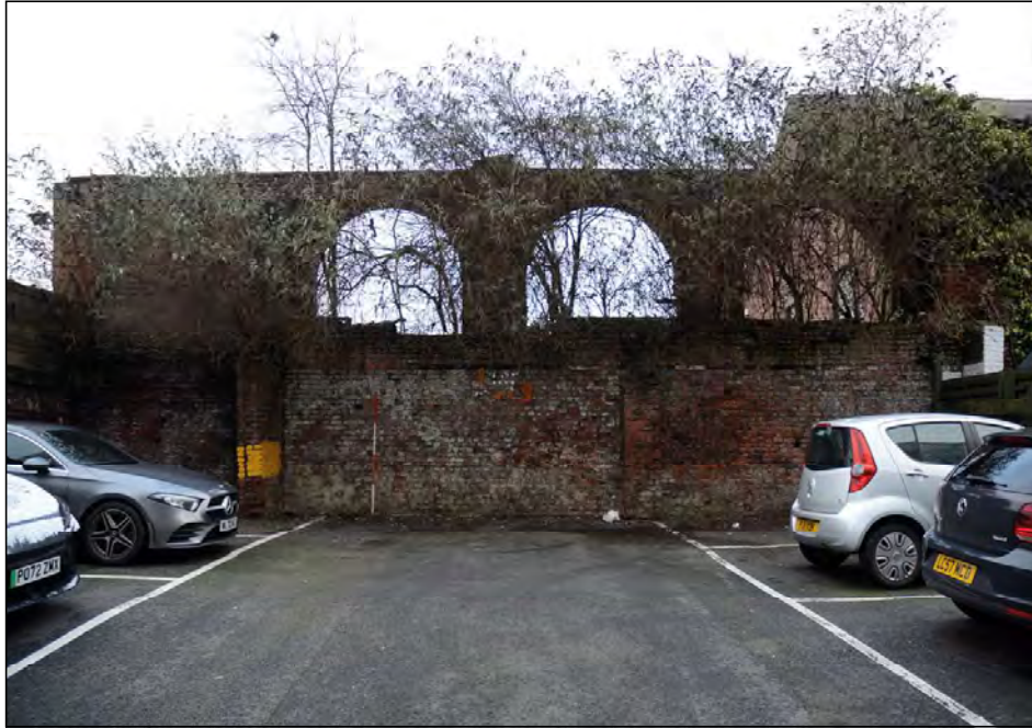
Plate 11. External arched wall of The Warehouse, looking east
