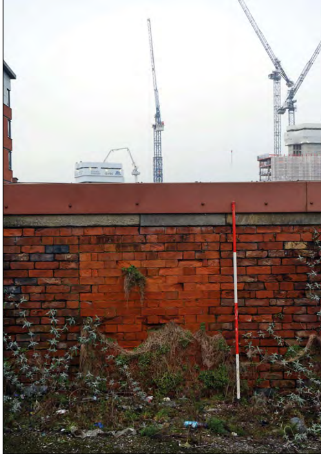
Plate 41. Blocked window of The Joiners Workshop, looking north
