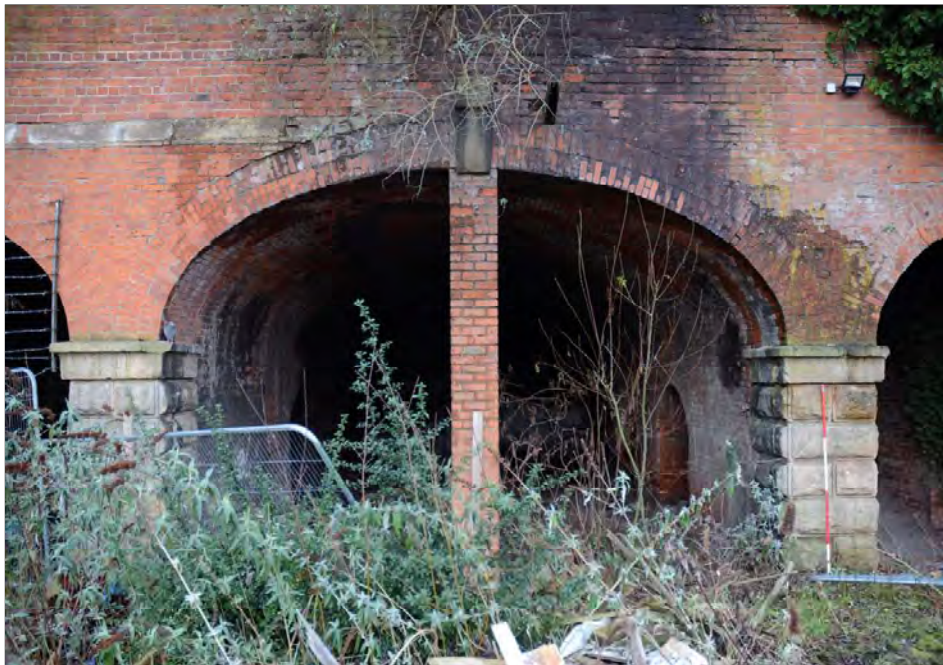
Plate 46. Detail of Cellar 3 arch, looking south
