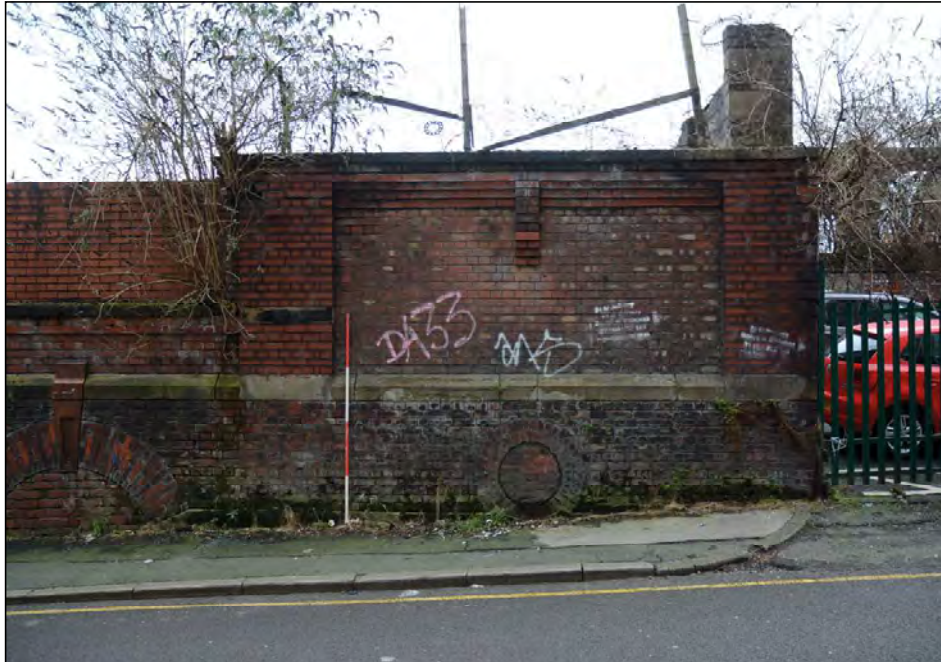
Plate 25. South-eastern corner of The Joiners Workshop, looking north
