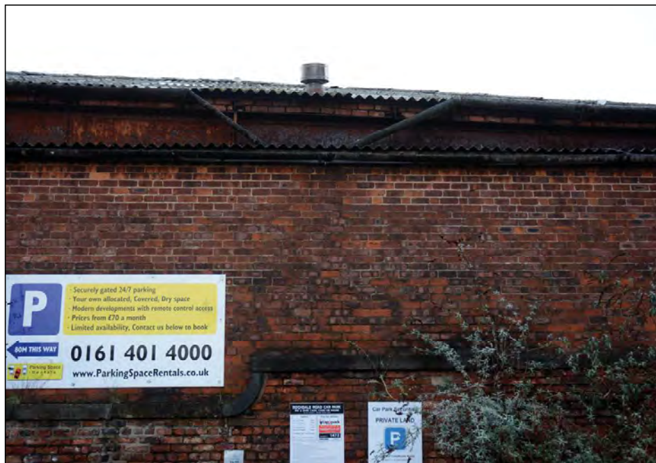
Plate 8. Inserted wall and roof, looking north
