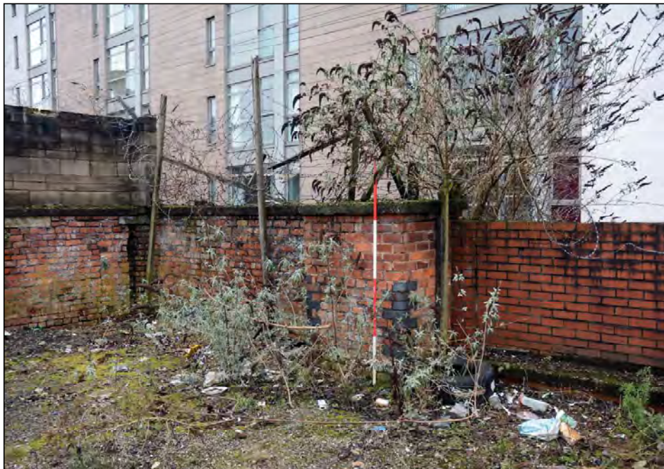
Plate 34. South-western corner of The Joiners Workshop, looking south-west
