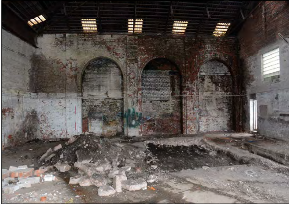
Plate 9. Internal western elevation of The Warehouse, looking west
