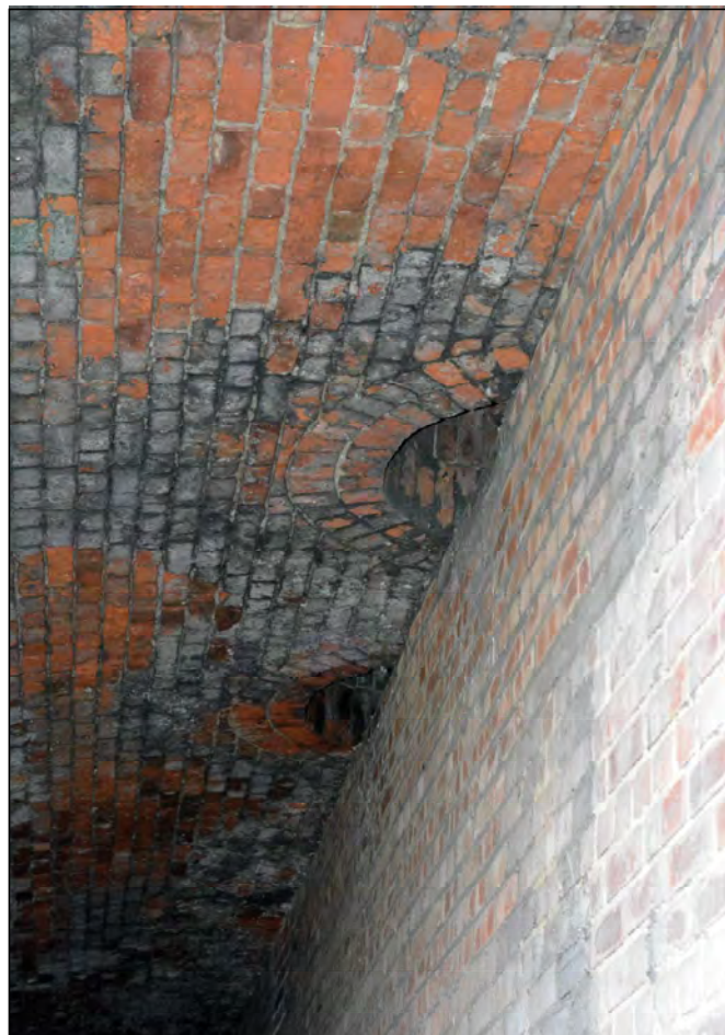
Plate 56. Brick chutes in Cellar 3, looking south
