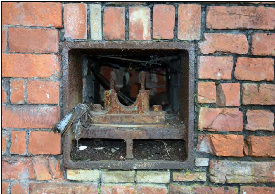
Plate 40. Detail of line shaft bearing box, looking north
