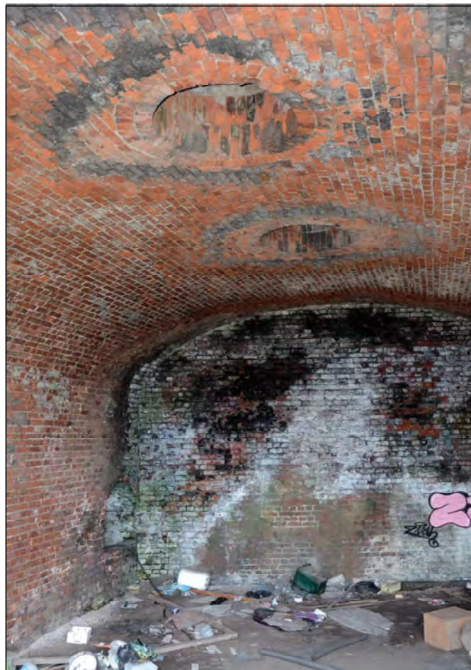
Plate 50. Cellar 1, looking south
