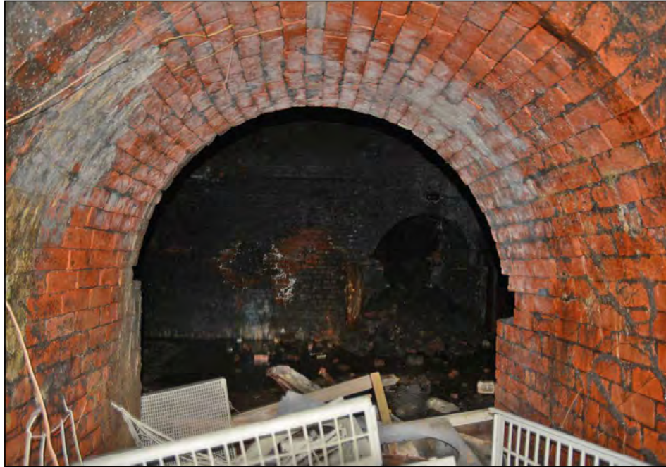
Plate 65. View of cellar tunnel, looking south
