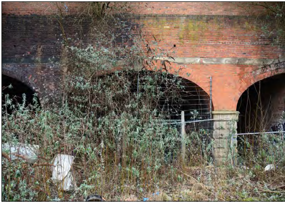
Plate 52. Cellar 2, looking south
