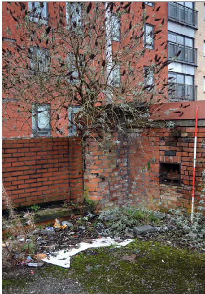
Plate 35. North-western corner of The Joiners Workshop, looking north-west
