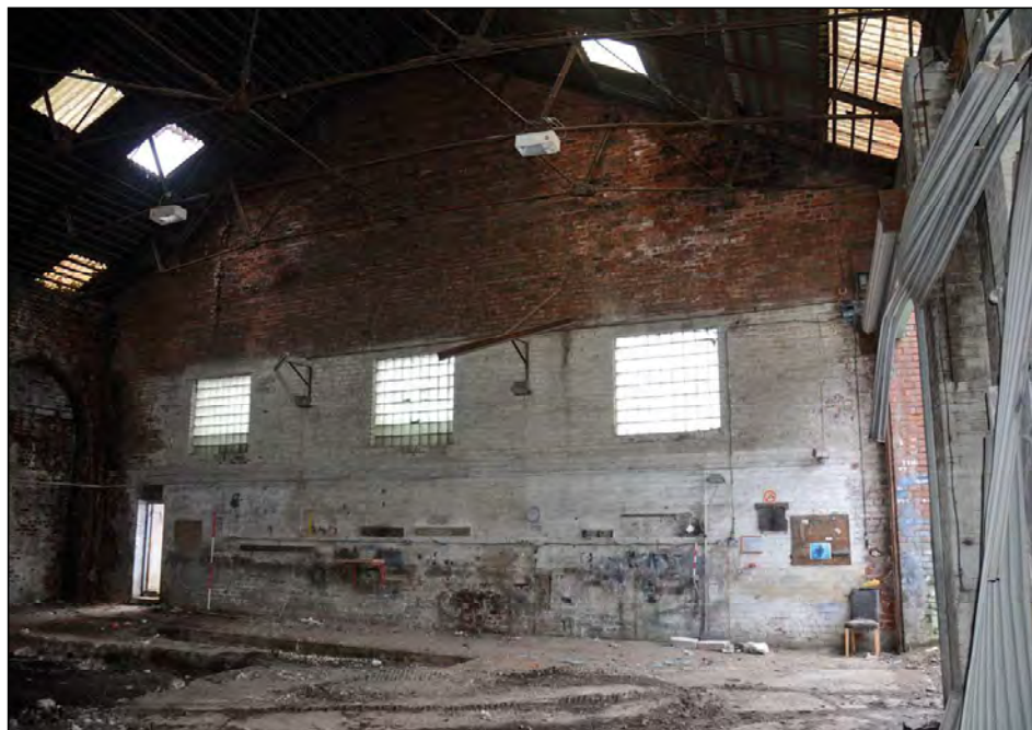
Plate 20. Later 20th-century wall inserted into The Warehouse, looking north-west
