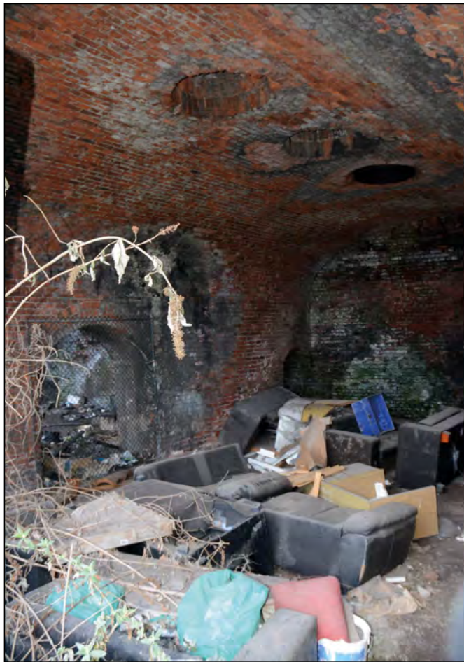
Plate 53. Cellar 2, looking south-east
