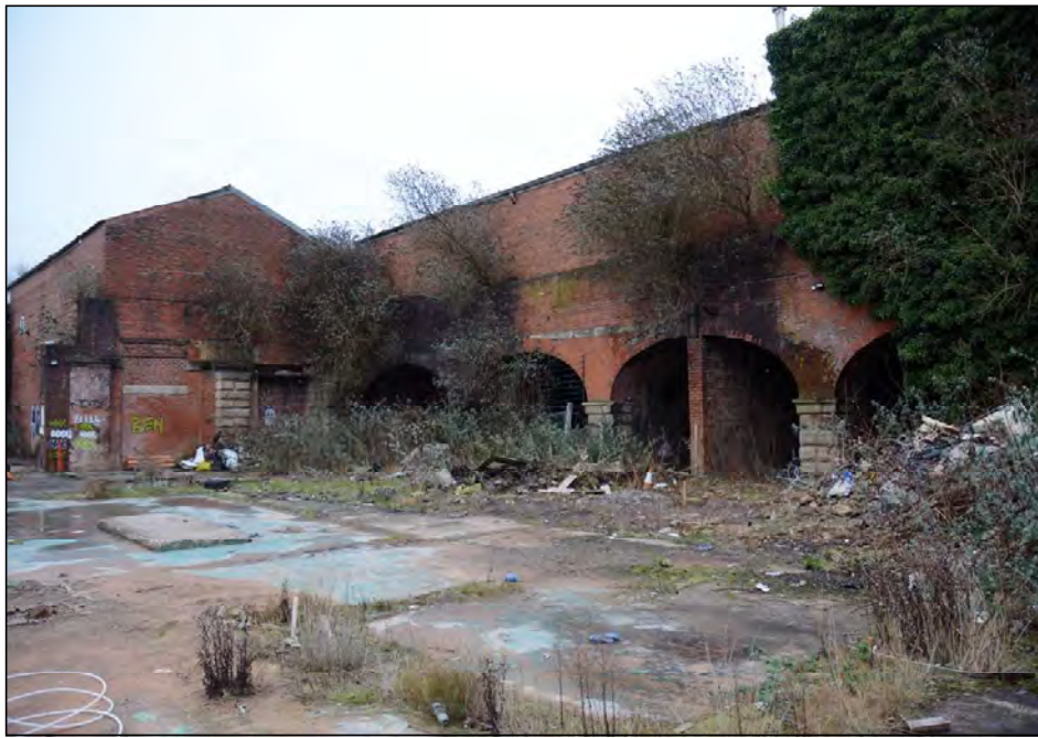
Plate 44. General view of eastern arches, looking south-east
