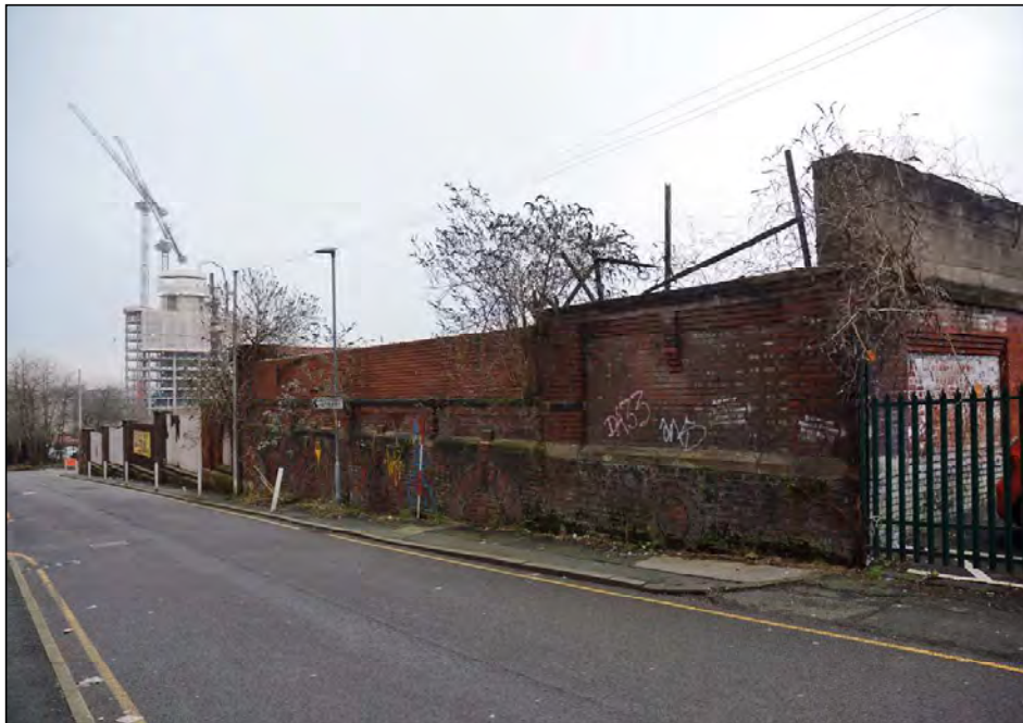
Plate 30. Western external elevation of The Joiners Workshop, looking north-east
