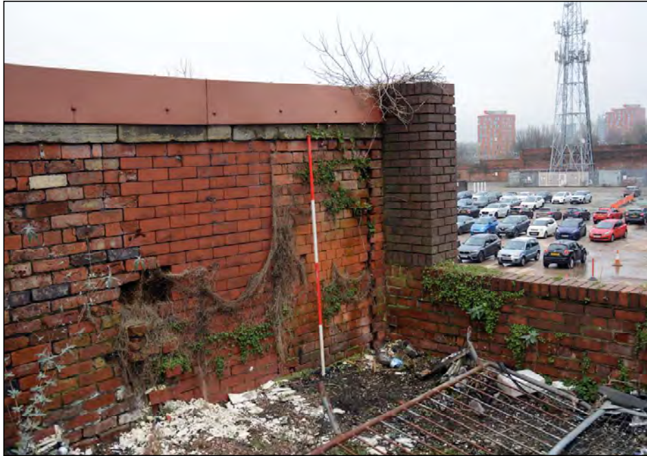
Plate 43. Blocked window of The Joiners Workshop, looking north
