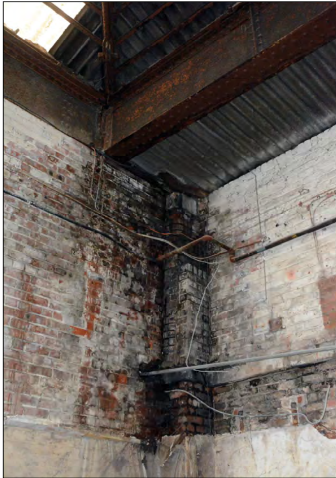
Plate 17. South-eastern corner of The Warehouse showing the iron beam and roof extension, looking south-east
