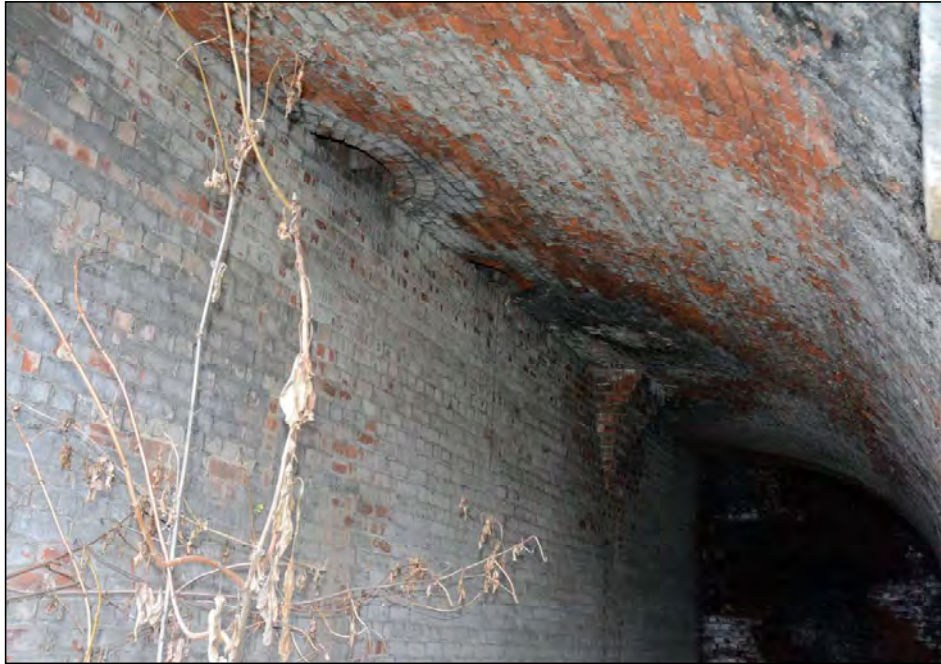
Plate 57. Cellar 3, looking south-east
