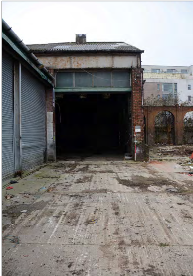
Plate 21. Eastern external elevation of The Warehouse, looking west
