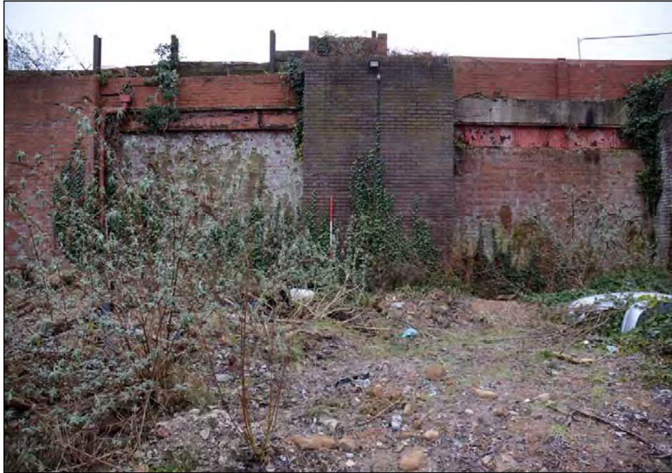
Plate 67. Beam 2 and 3, looking south
