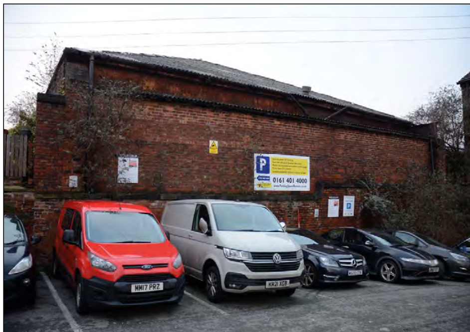
Plate 5. Southern external elevation of the Warehouse, looking north
