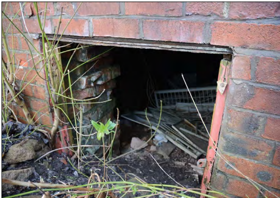
Plate 64. Entrance into cellar tunnel, looking south
