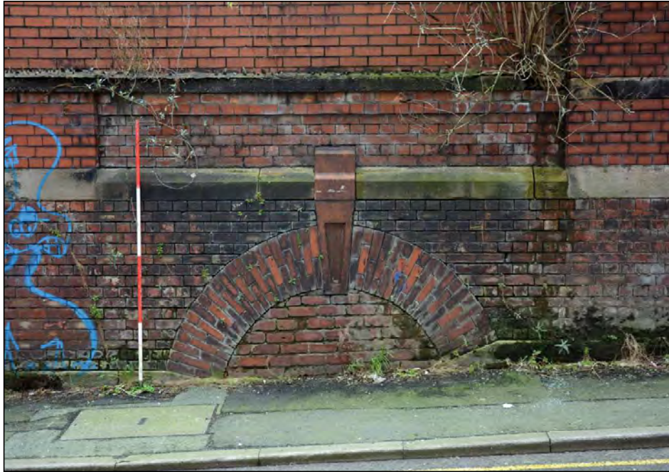
Plate 37. Arched blocked window of The Joiners Workshop, looking west
