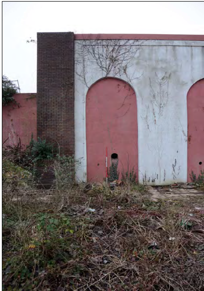
Plate 70. Detail of one of the western arches, looking south
