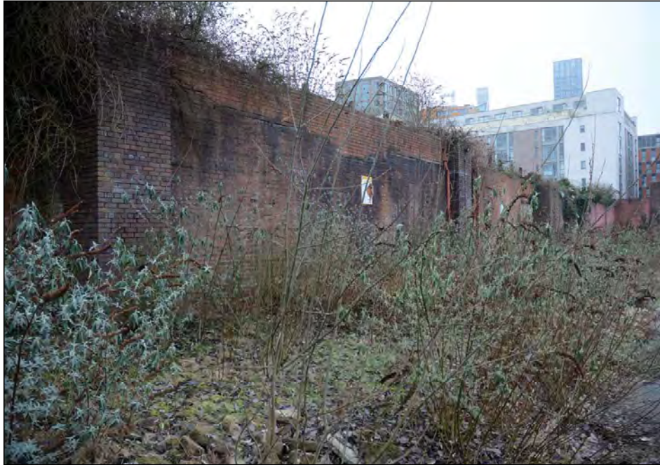
Plate 63. Later 20th-century brick work buttressing the northern wall, looking south-west
