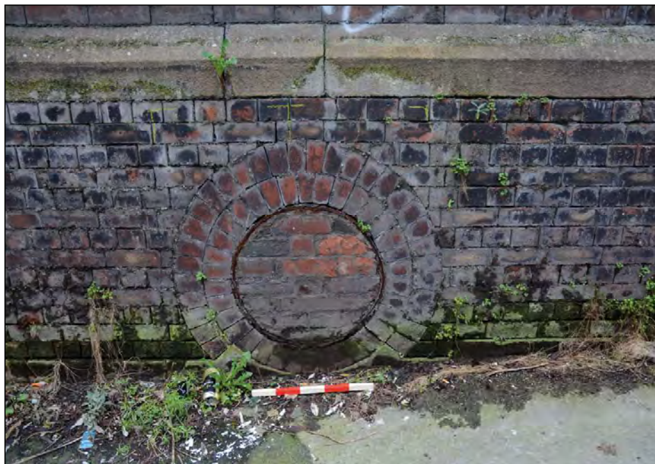
Plate 36. Round blocked window of The Joiners Workshop, looking east
