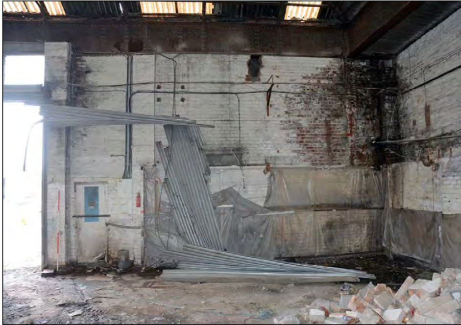
Plate 23. Eastern internal elevation of The Warehouse, looking east
