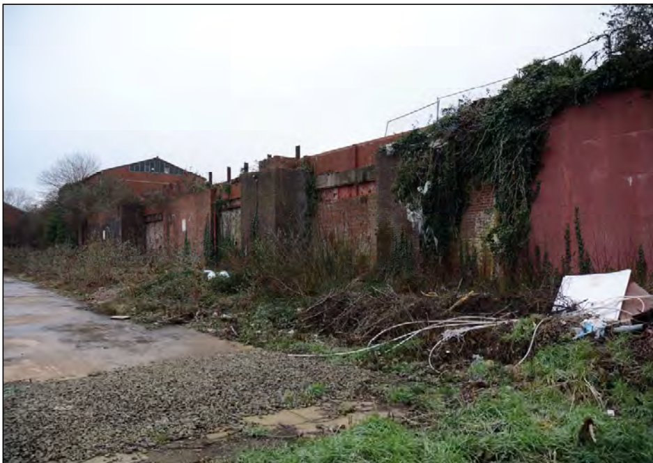
Plate 62. General view of Northern Wall looking south-east
