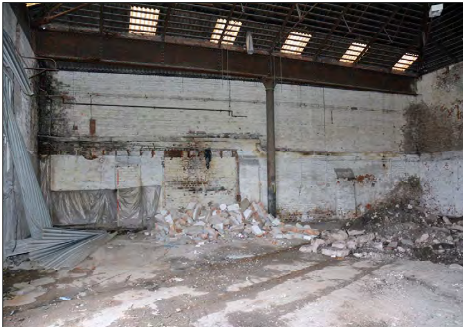
Plate 4. Southern internal elevation of The Warehouse, looking south
