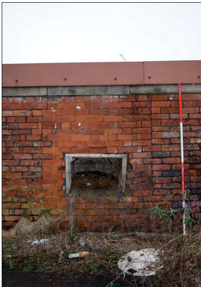
Plate 42. Blocked window of The Joiners Workshop, looking north
