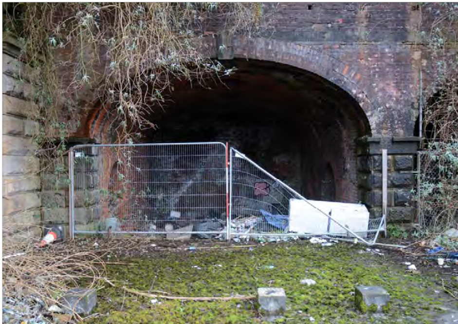
Plate 48. Cellar 1, looking south
