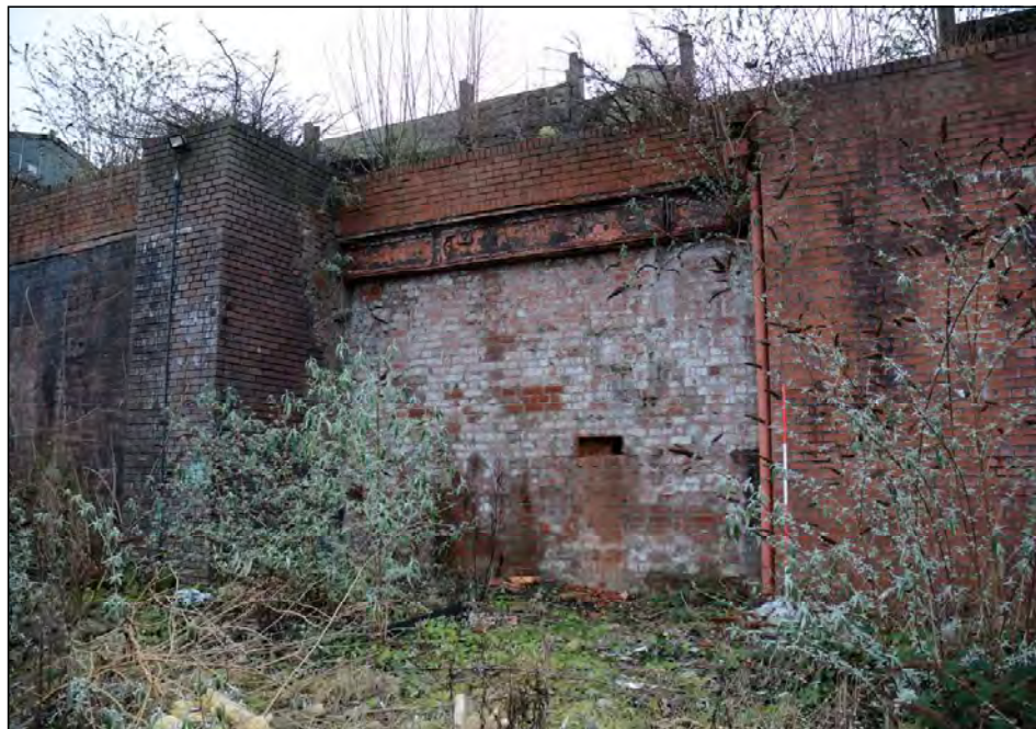
Plate 66. Beam 1, looking south-east
