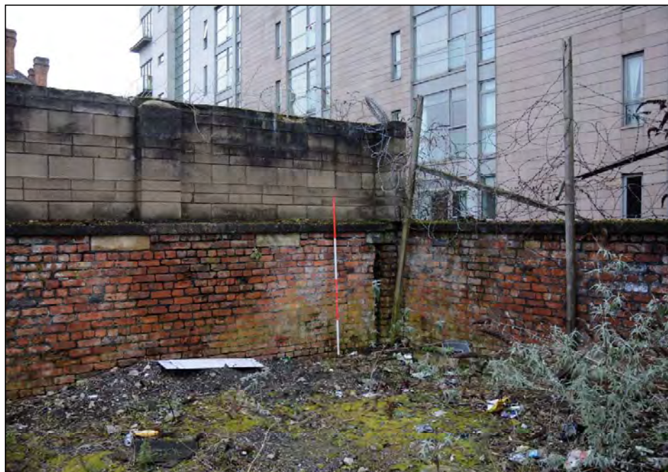
Plate 28. South-western corner of The Joiners Workshop, looking south-west
