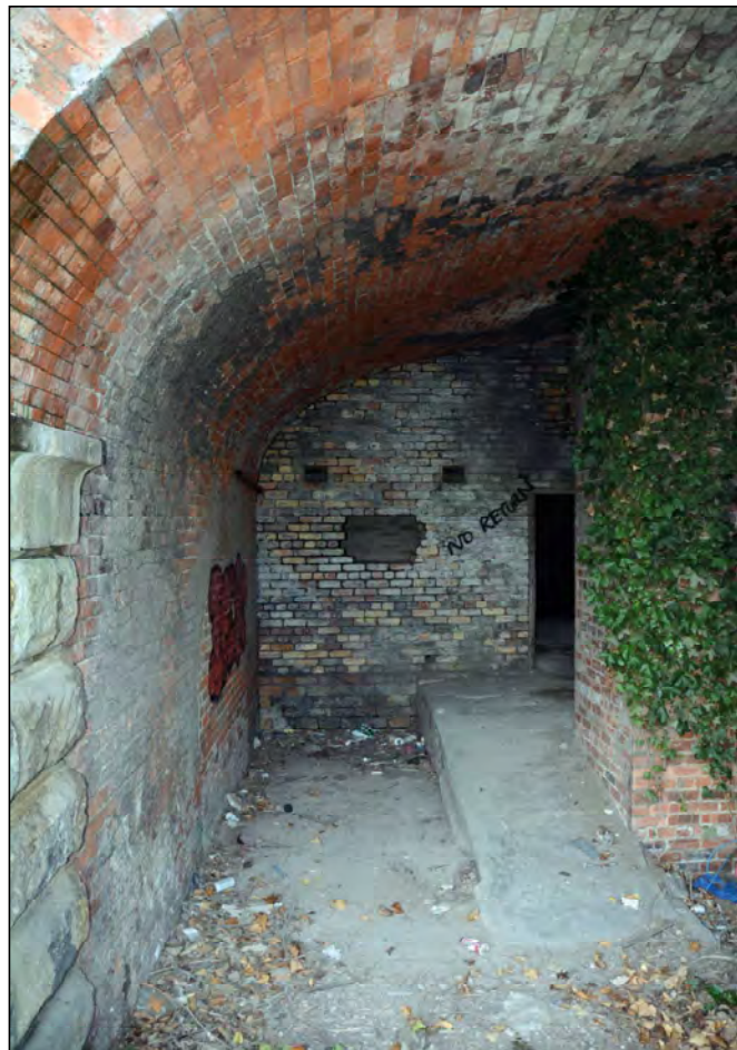
Plate 60. Cellar 4, looking south
