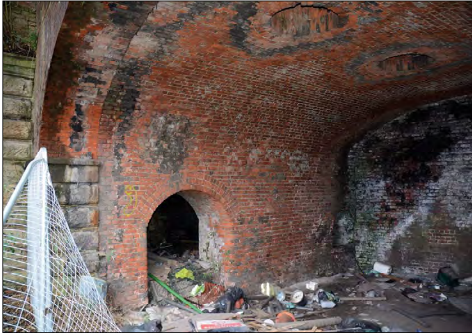
Plate 49. Cellar 1, looking south-east
