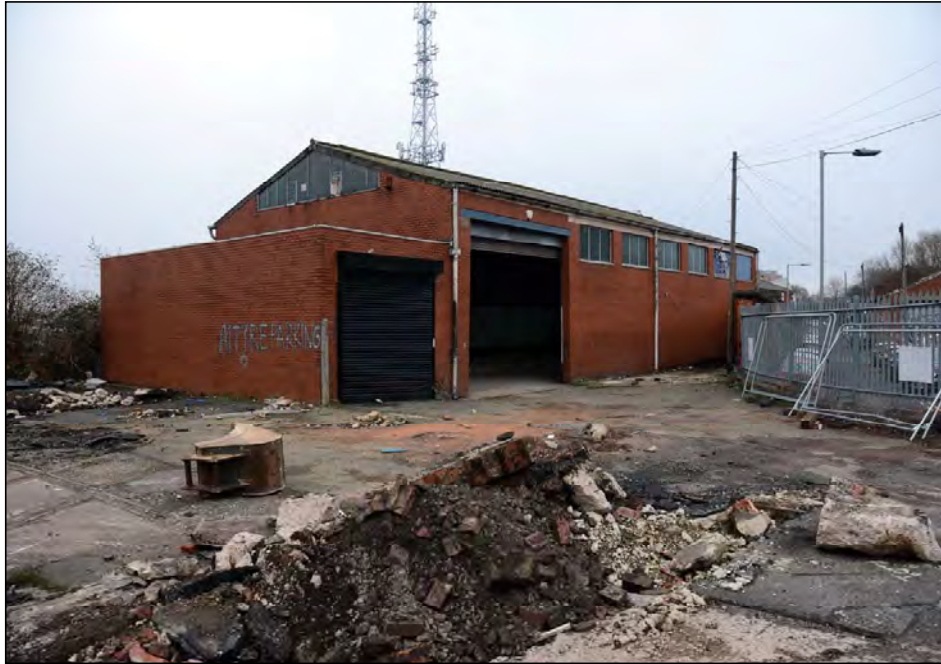
Plate 3. Later 20th-century depot, looking north-east
