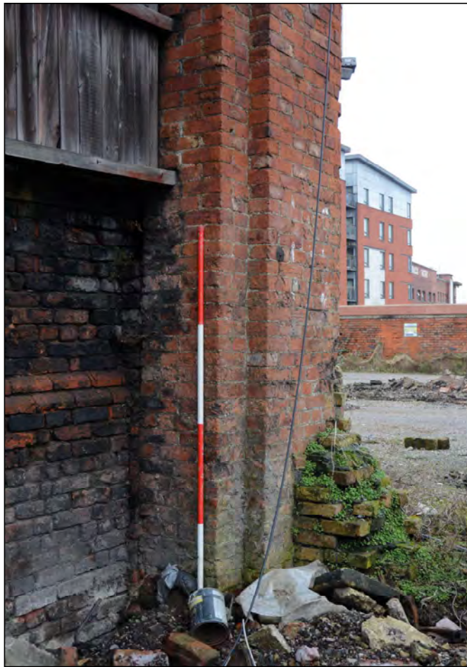
Plate 29. Overlapping walls of The Joiners Workshop and Warehouse, looking north-west
