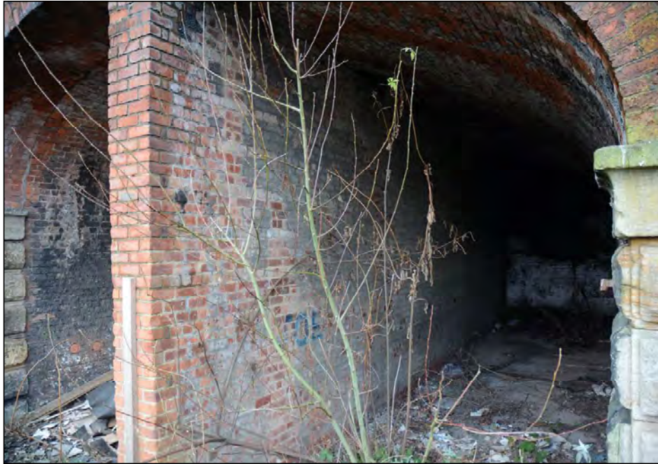
Plate 55. Cellar 3 dividing wall, looking south-east
