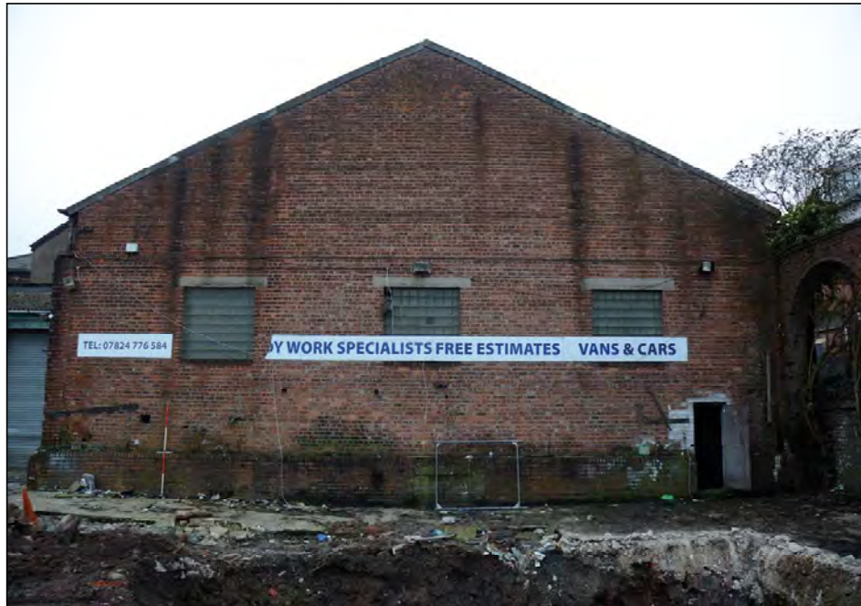
Plate 19. Later 20th-century wall inserted into The Warehouse, looking south
