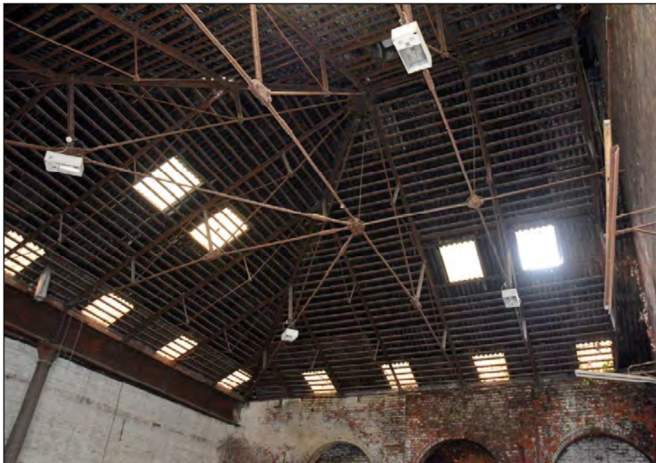
Plate 18. General view of The Warehouse roof, looking south-west
