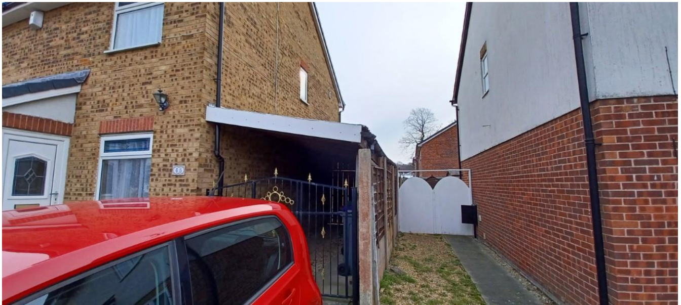
Figure 2. Front view of the proposed site of development.
