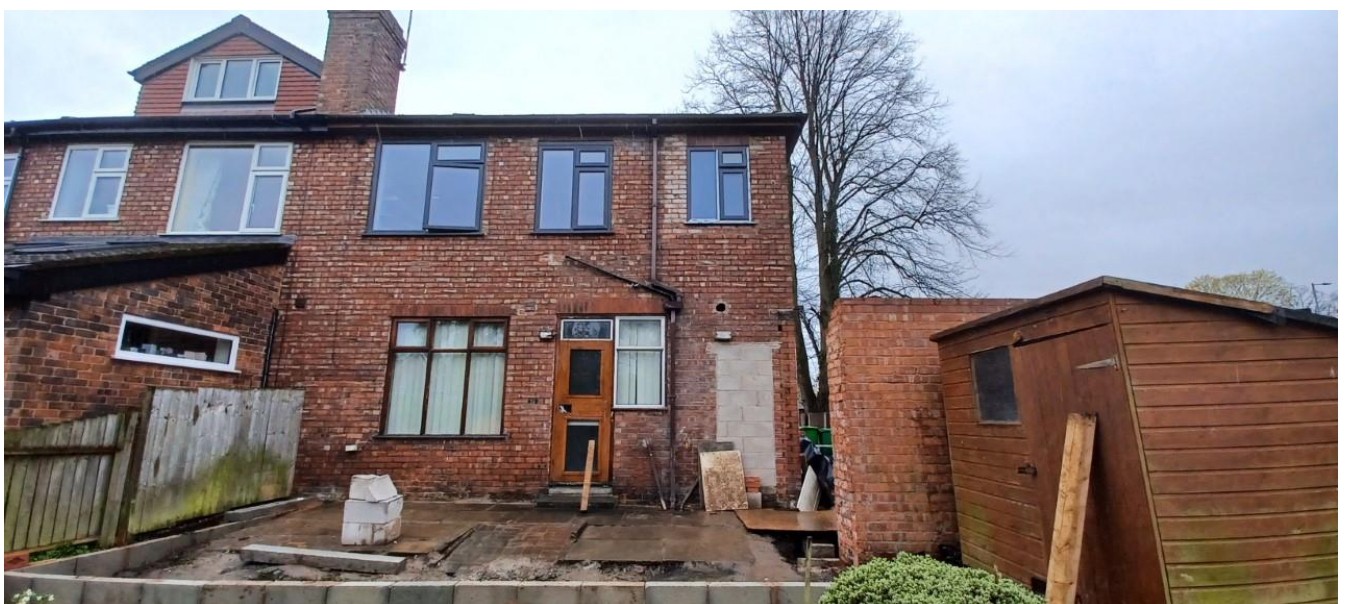
Figure 4. Rear view of property.
