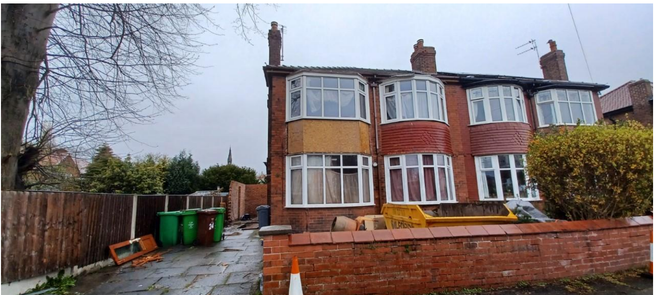
Figure 1. Principal elevation of No.24 Waltham Road.
