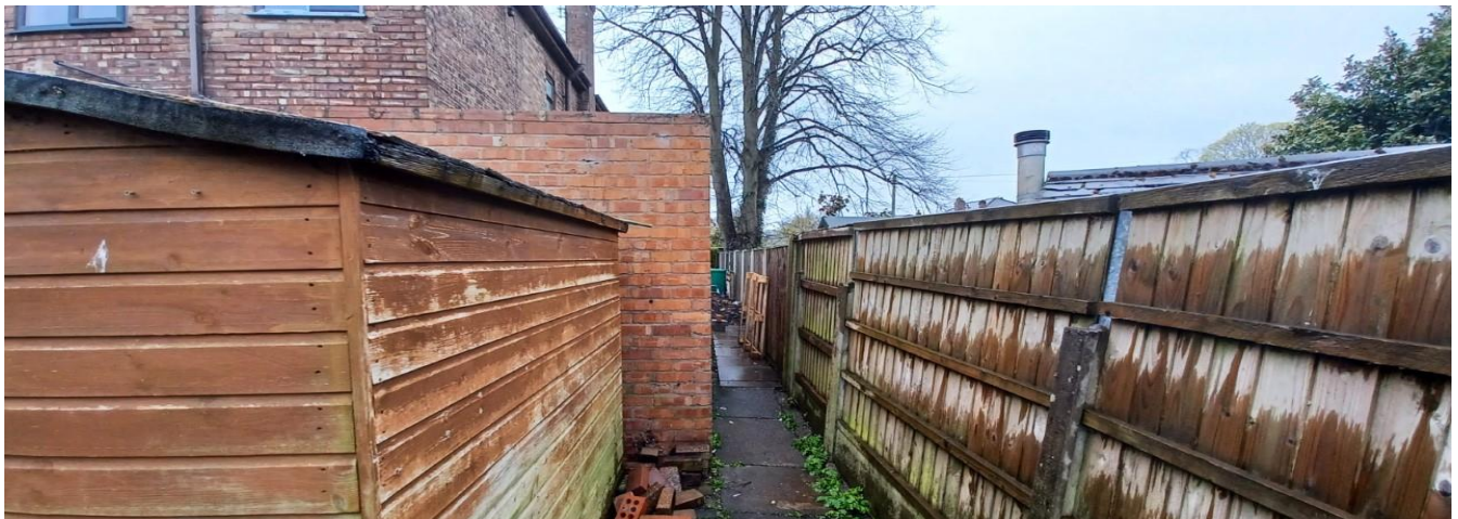
Figure 6. View of gap to shared boundary.
