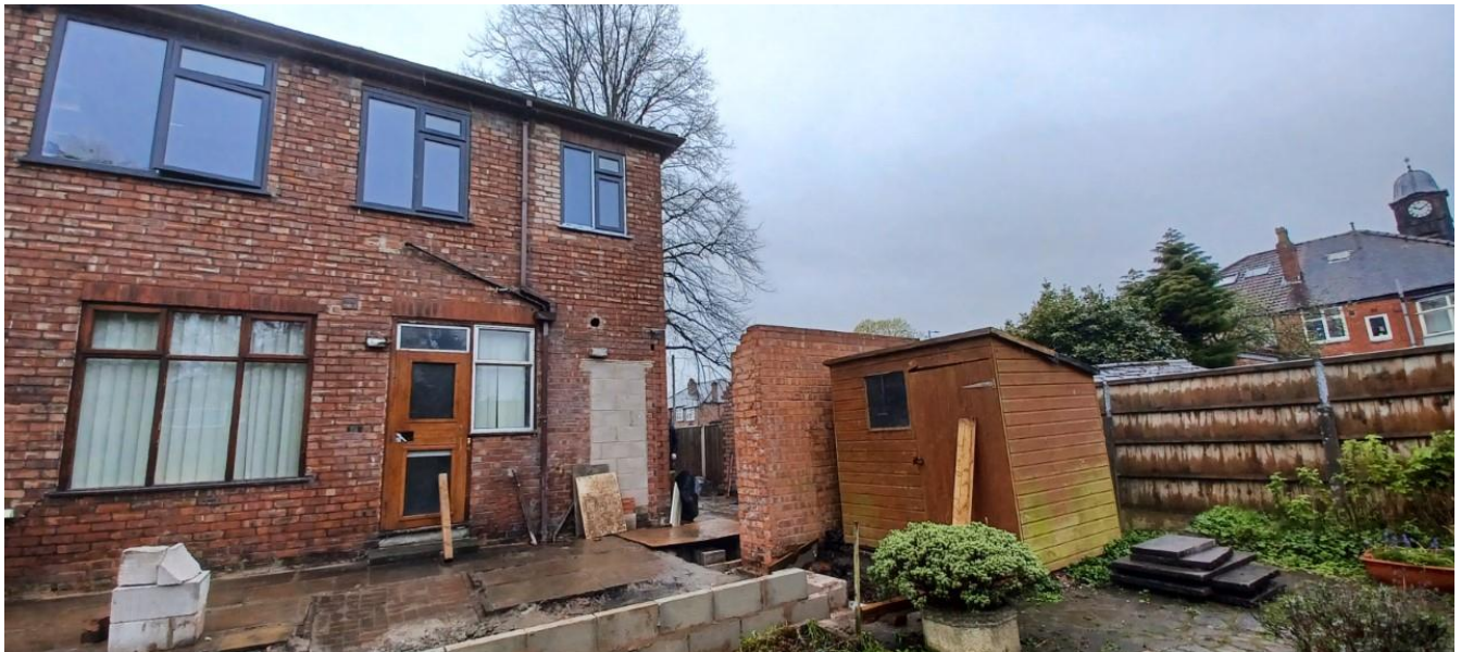
Figure 5. Rear view of property and its relationship with neighbouring properties along Alexandra Road South.
