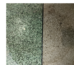
Assumed extent of terrazzo following exposed areas
