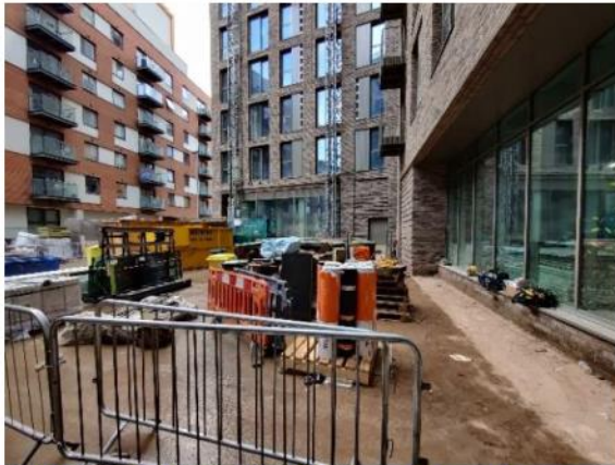
Figure 1: Ground floor not yet completed
