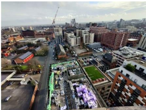
Figure 3: Aerial view of Floor 9 and 7 from Floor 15
