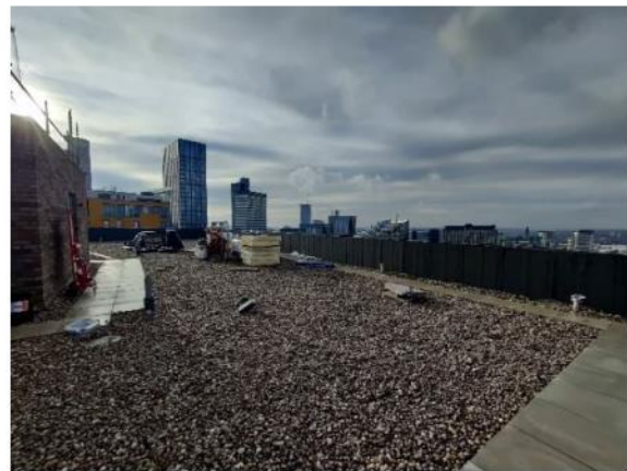
Figure 4: Floor 15 Stone ballast area for solar panel installation
