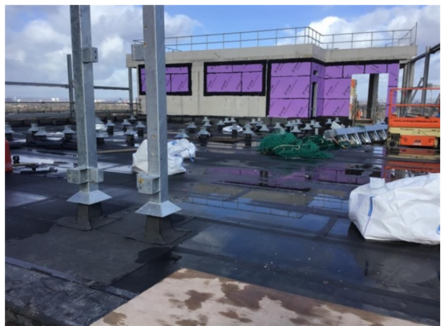
Photo 2 - View of progress to section 3
