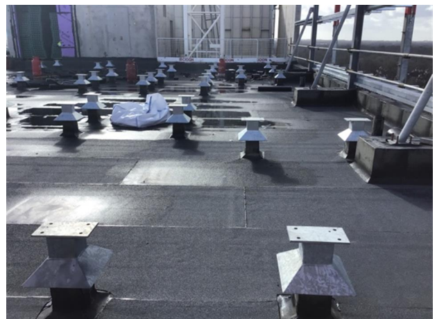
Photo 8 - View of cap sheet to section 3
