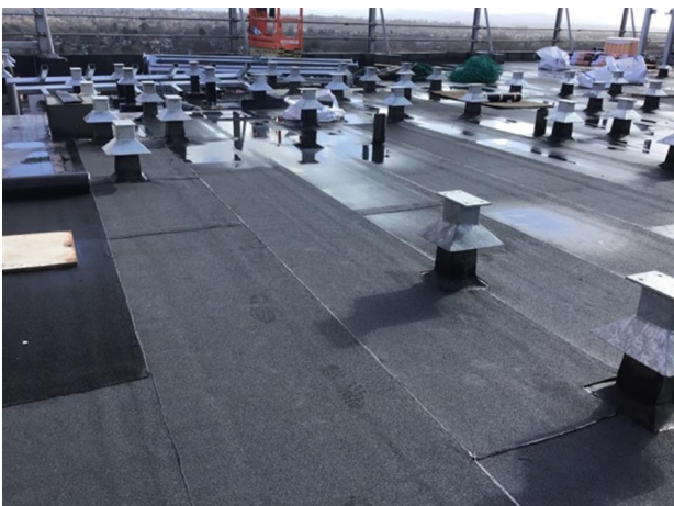
Photo 7 - View of cap sheet to section 3
