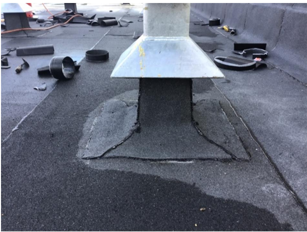
Photo 11 - View of cap sheet to posts
