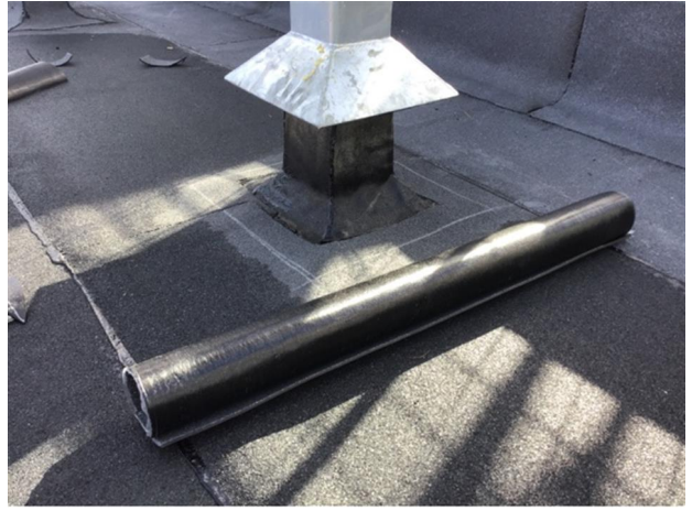
Photo 10 - View of second underlay layer to steel posts
