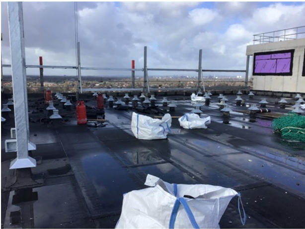
Photo 3 - View of progress to section 3
