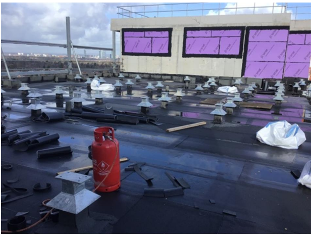
Photo 13 - Overview of level 9 section 3
