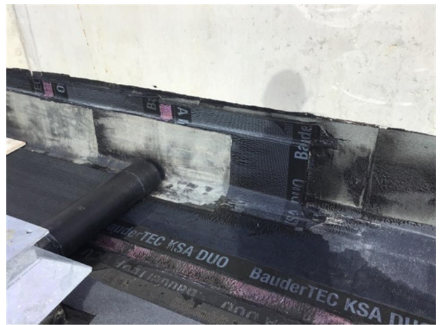
Photo 6 - View of build up to up stands
