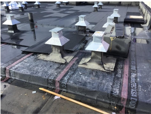
Photo 5 - View of second underlay layer to steel posts
