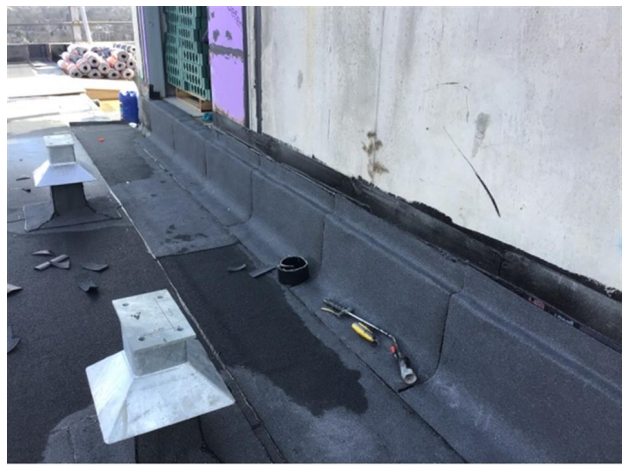
Photo 12 - View of cap sheet to up stand
