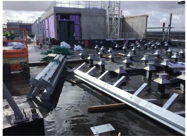
Photo 4 - Overview of section 3
