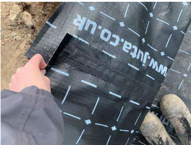
Figure 3 – Correct auto-welding.
