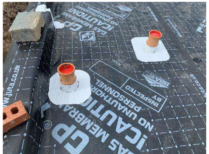
Figure 4 – Service penetrations sealed using detailing strip.
