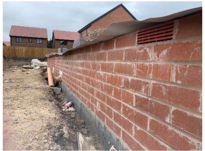
Figure 2 – Air bricks installed at 2m centres.
