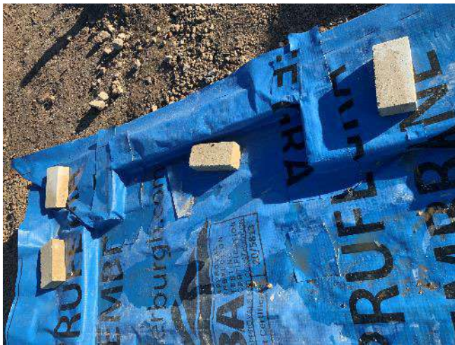
Figure 13 – Corners formed correctly using double sided tape.
