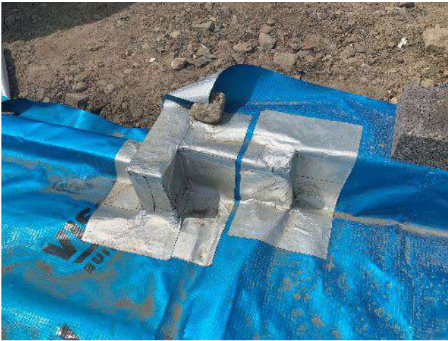
Figure 5 – Corners installed using detailing strip.
