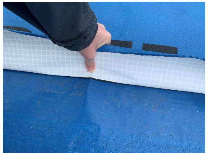
Figure 10 – Correct jointing with double sided tape.
