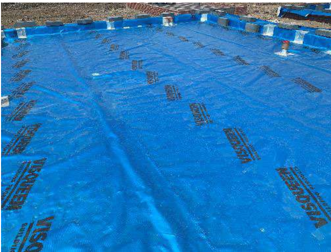
Figure 7 – Membrane kept free of stones, debris and equipment to ensure it stays intact. No holes, tears or punctures are present.
