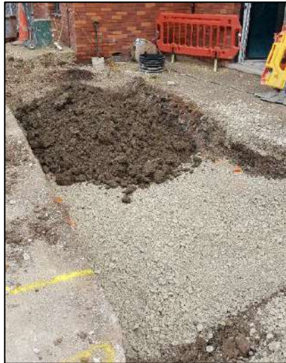
Figure 3: The break layer is overlain by 300mm sub-soil, seen here before spreading across the garden:
