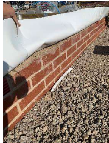
Figure 8 – Sufficient overlap of cavity.
