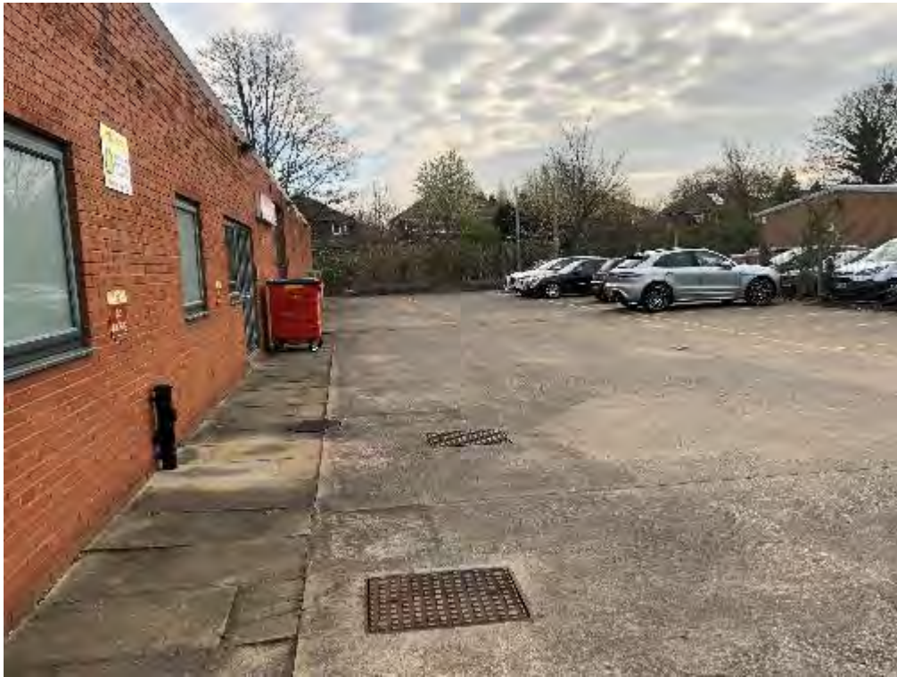
PLATE 5 CAR PARKING IN SOUTH OF SITE
