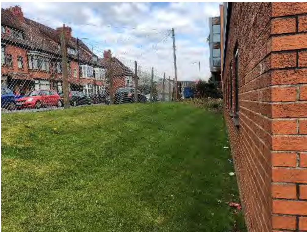
PLATE 4 EMBANKMENT ON WESTERN BOUNDARY
