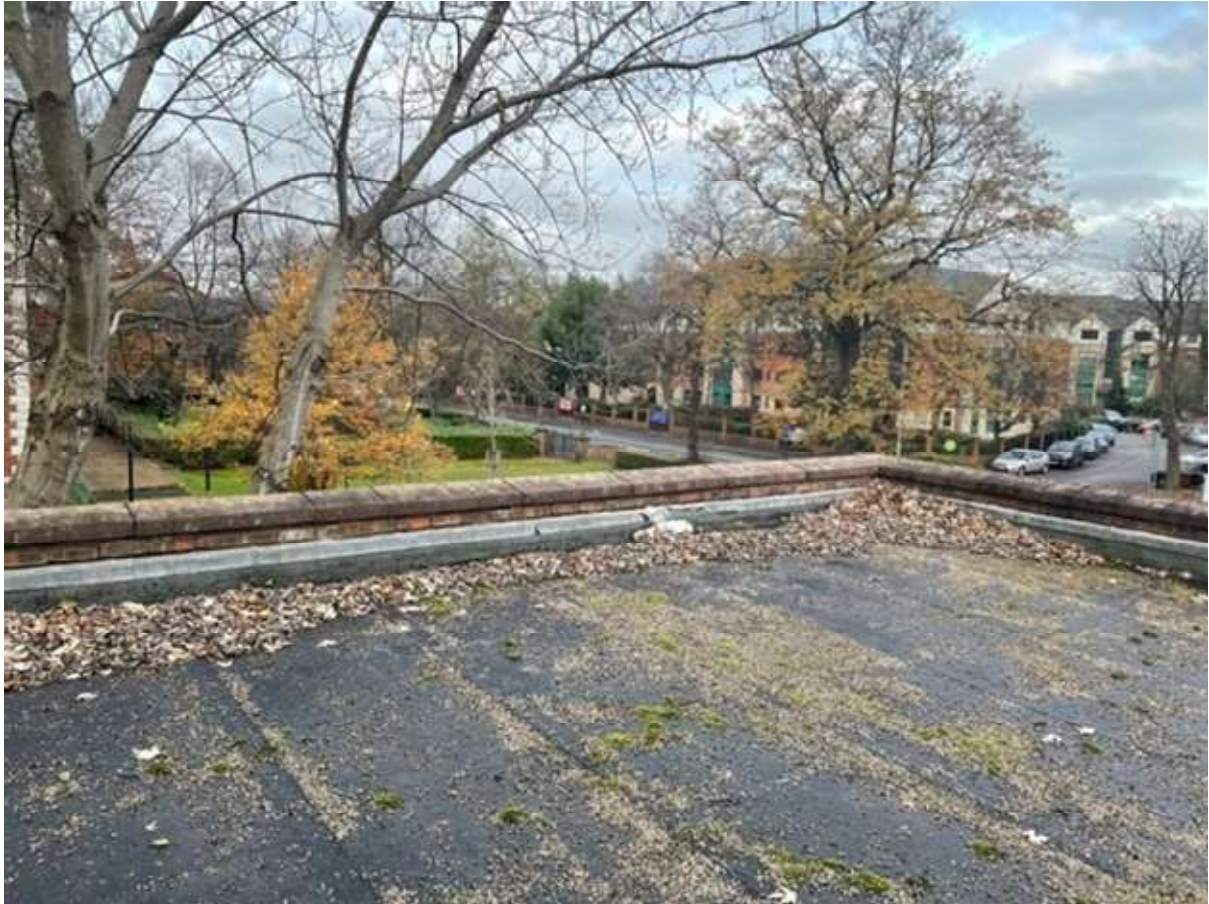
Photo 4. Existing roof covering, showing lead flashing upstand detail and parapet wall.
