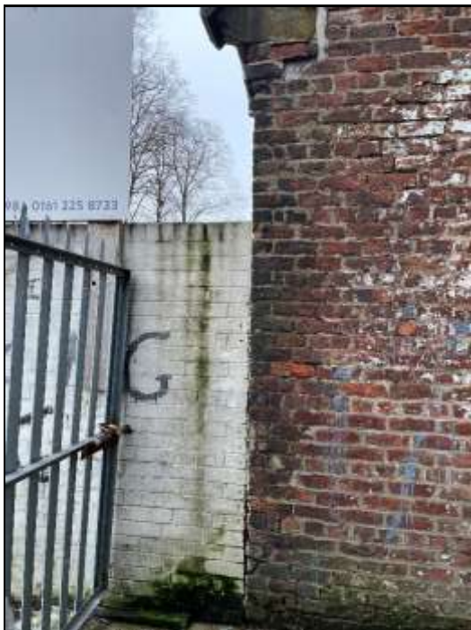
Photograph 2 – Existing gable wall of the Parish Hall and non-original boundary wall abutting the same viewed from Walmer Street East.
