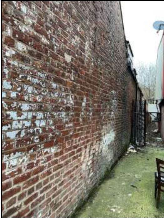
Photograph 1 – Existing gable wall of the Parish Hall viewed from Walmer Street East
