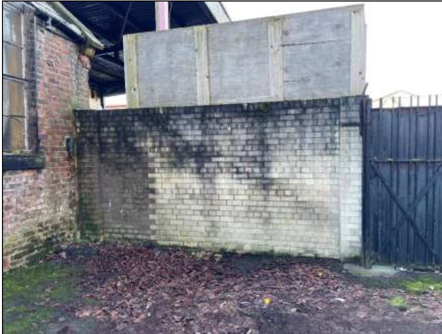
Photograph 3 – Existing boundary wall with Walmer Street East viewed from within the Parish Hall site on the reverse side of photograph 2.
