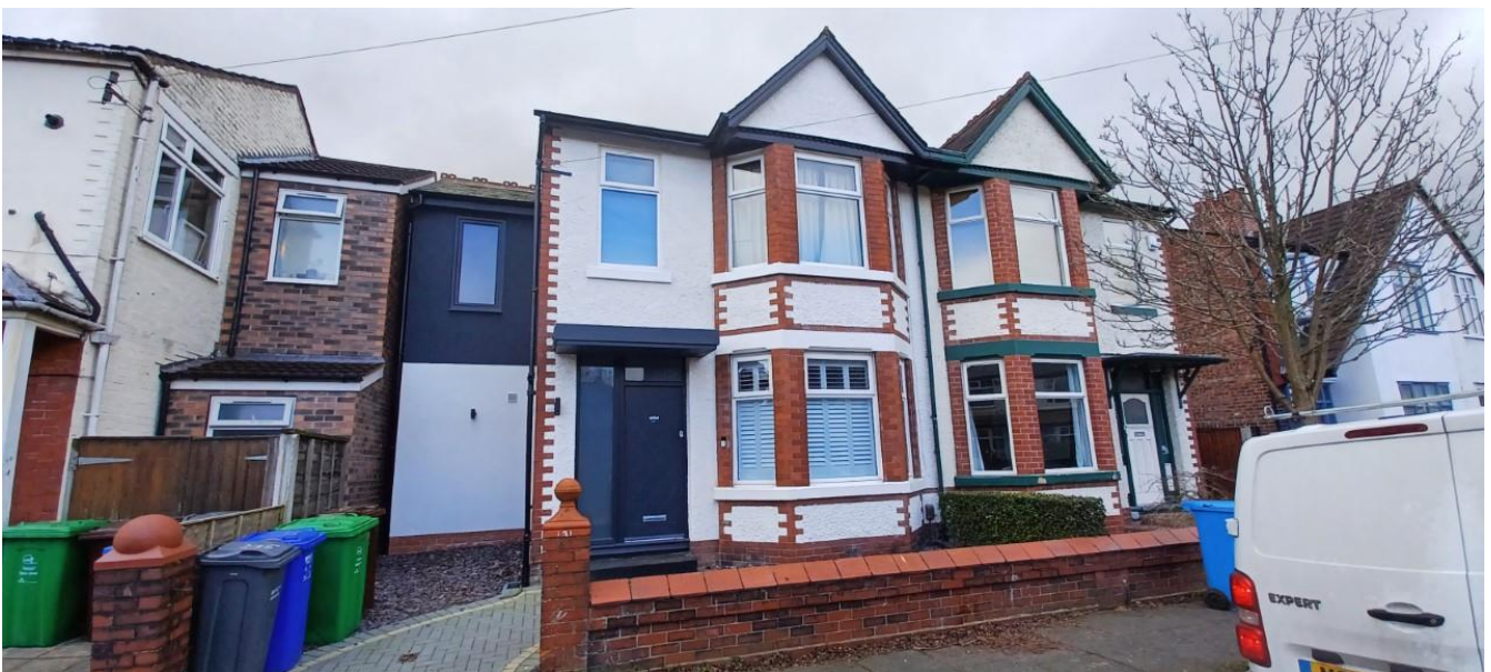
Figure 1. Principal elevation of No.121 Newport Road.
