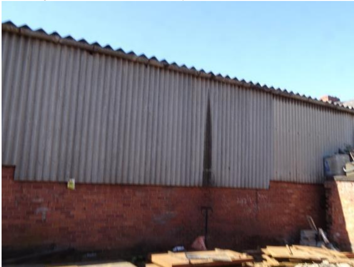
The building to the west of the site and western yard
