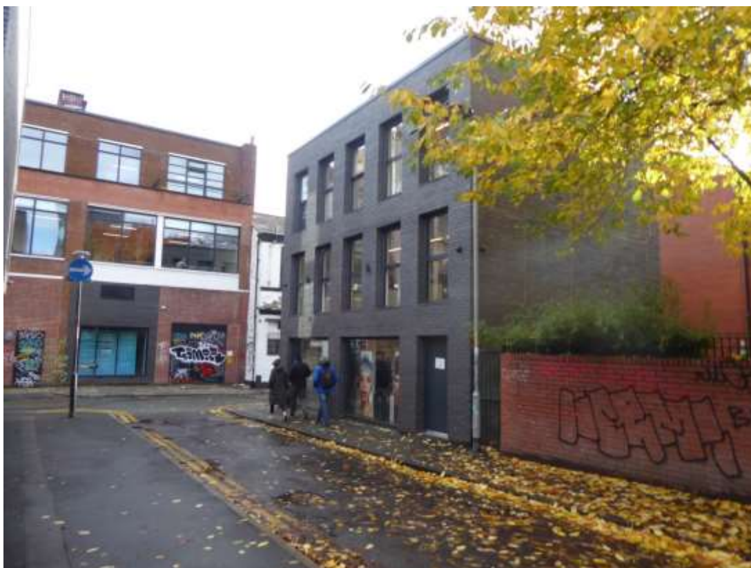
Fig 2. View of Side and Rear Elevation from Foundry Street
