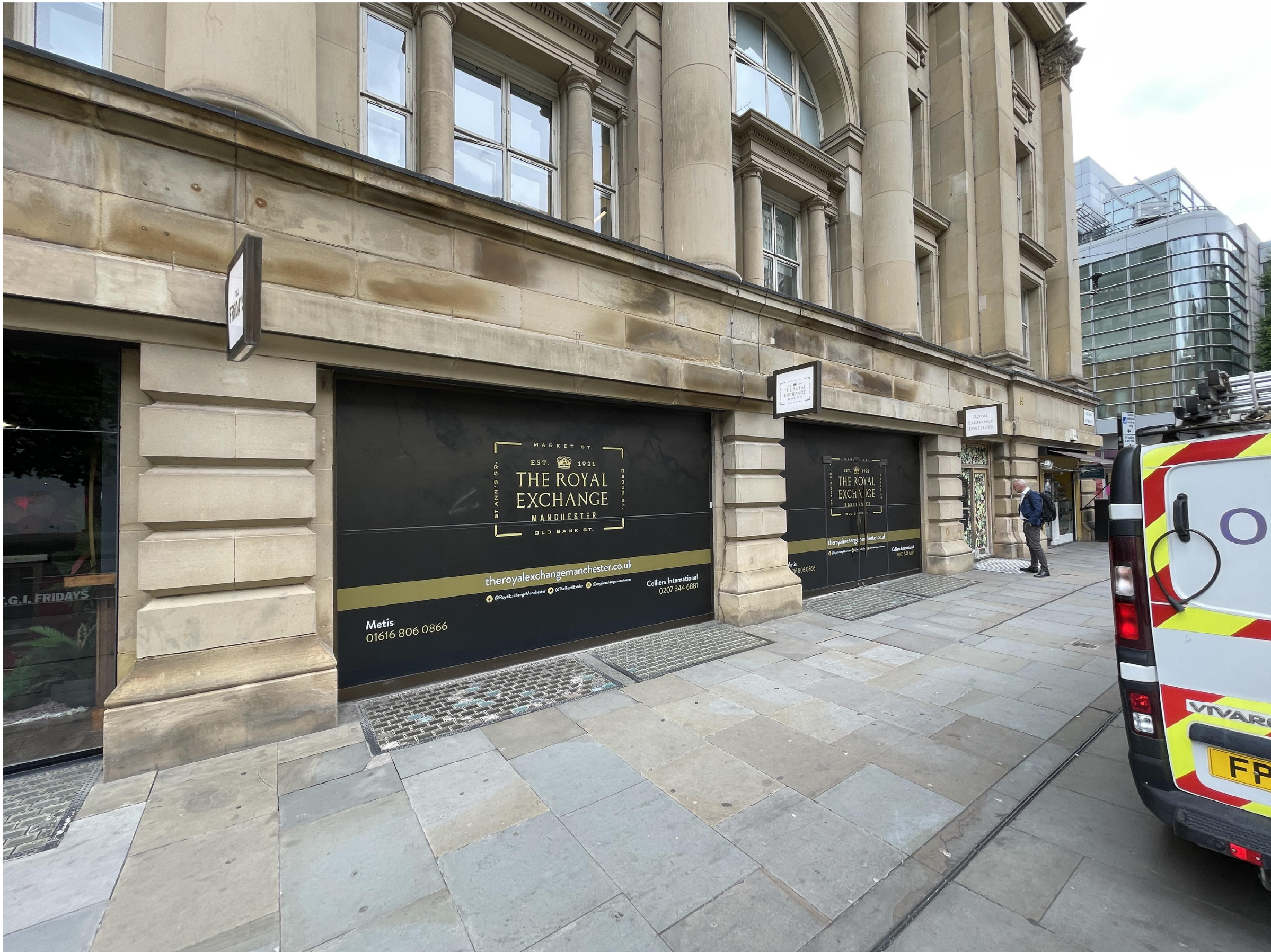
Existing views of store front facing cross street
