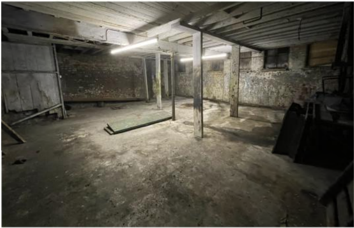
The basement floor is non-original concrete slab which dishes towards central low point and floor gulley. Another floor gulley is present in the rear corner.
